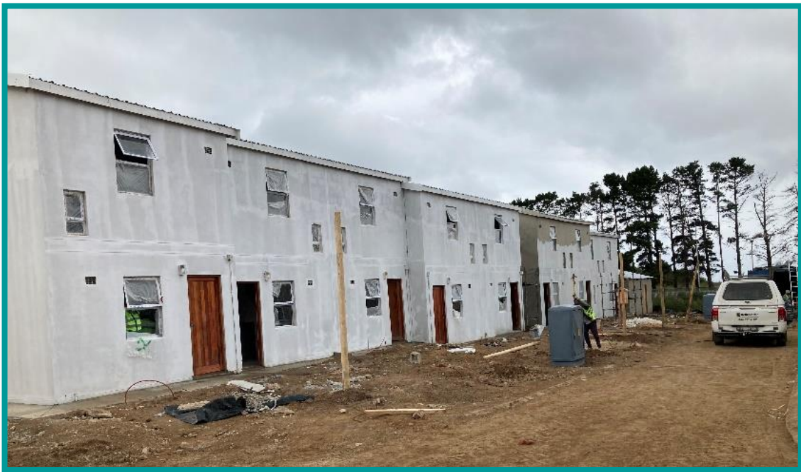
Picture 1: Construction of Qolweni/Bossiesgif 169
