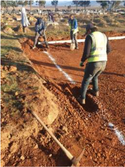
12 May 2022 – The first trenches for the Driving Test Range
