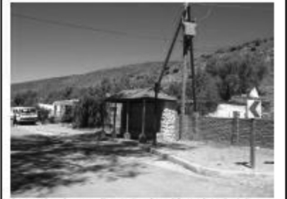
Example of upgrading using local found materials along Hoof Street
