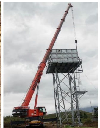
Installation of Suurbraak 150l water tank
