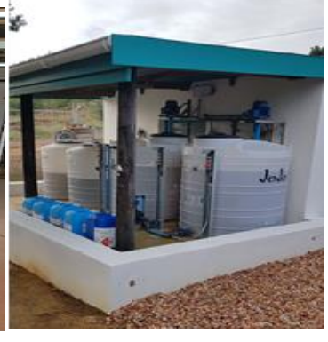
Upgraded dosing Building and equipment
