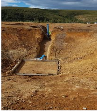
Construction work at gravity sump
