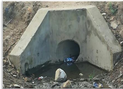
Buffeljagsrivier Storm Water Drainage
