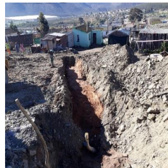
Barrydale Housing and infrastructure upgrading
