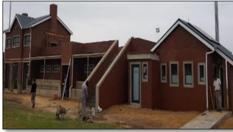
Railton Sports Stadium
