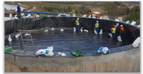
Barrydale bulk water Infrastructure. Phase 1
