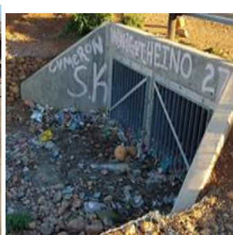
Culvert in Angelier Street
