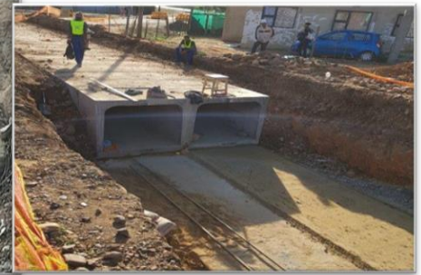
Railton upgrade gravel roads and storm water phase 2
