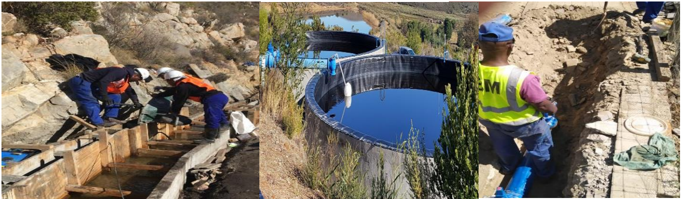
Phase 1 of the Barrydale Bulk Services: Housing Project.
