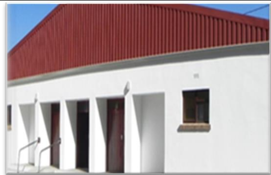
Upgrading of Suurbraak community Hall.- 23 March 2018.
