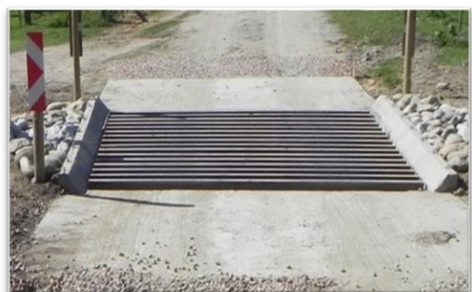
Construction of 3 Cattle Grids, Gates and Fencing
