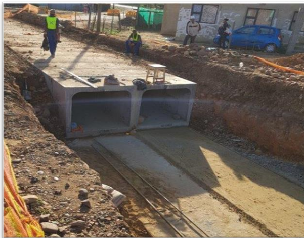
Railton upgrade gravel roads and storm water phase 2
