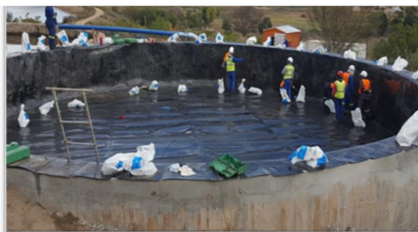
Upgrade Phase 1 Barrydale bulk water Infrastructure by 30 June 2018
