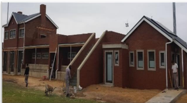
Complete Phase 2 of the Railton Sports Stadium upgrade by 30 June 2018
