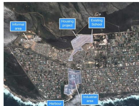
Figure 15: Kleinmond integrated housing development
