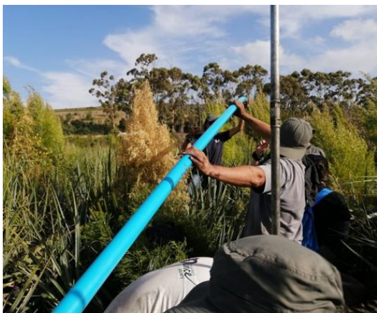
Monitoring wells being installed.
