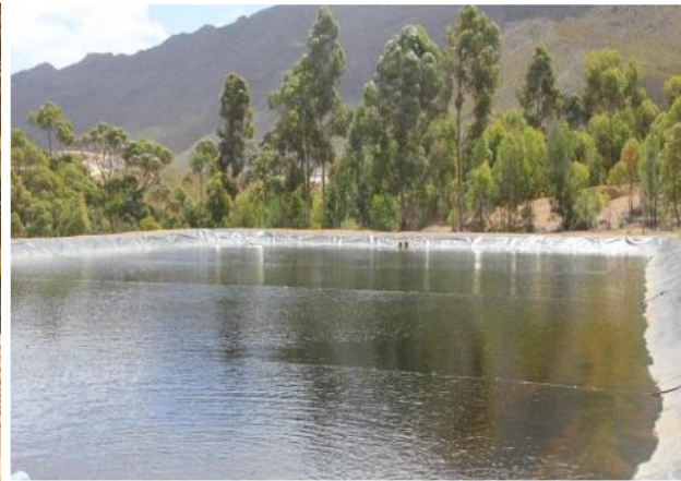
3 MI Storage dam for supply from Kommissiekraal, Elandskloof and boreholes
