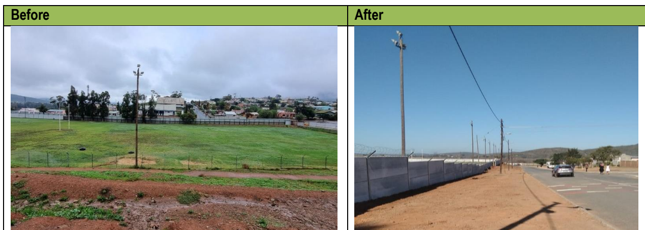
Photo: Precast Boundary Wall completed at Happy Valley Sportsground, Bonnievale
