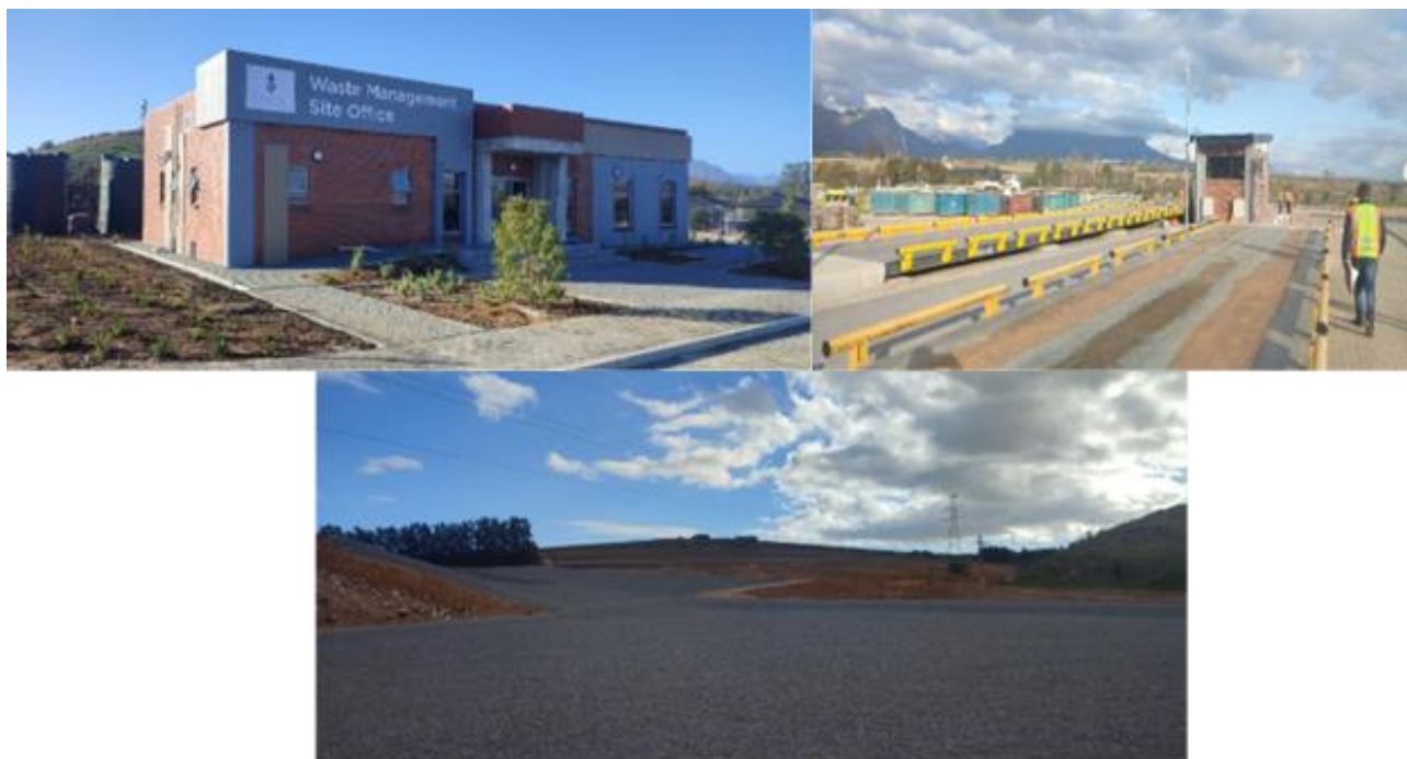
Stellenbosch Landfill New Cells and Associated Infrastructure
