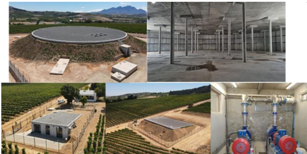
Construction of a new Reservoir and Pipeline: Vloottenburg – Phase 1 water will be provided to Polkedraai, Digtebij, Longlands and surrounding farms.
