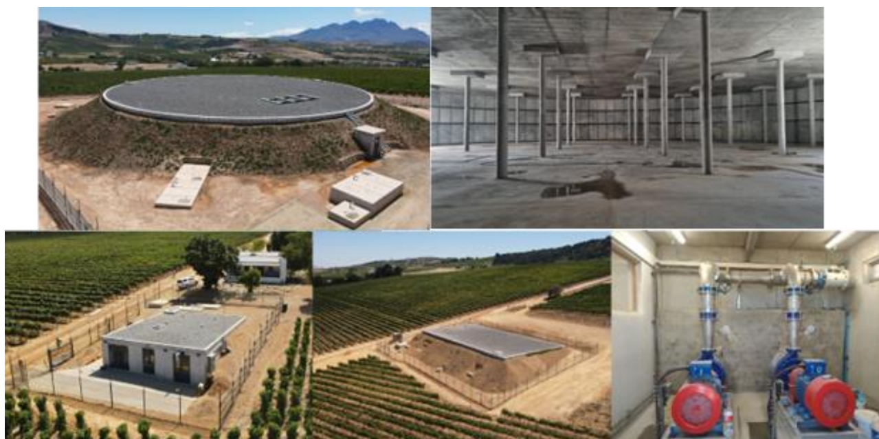
Vlottenburg New Reservoir, Pipeline and Associated Works
