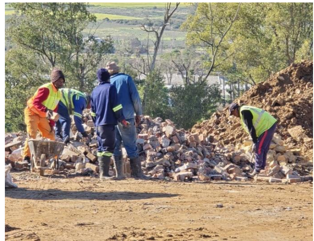
Reclaiming of bricks at the site
