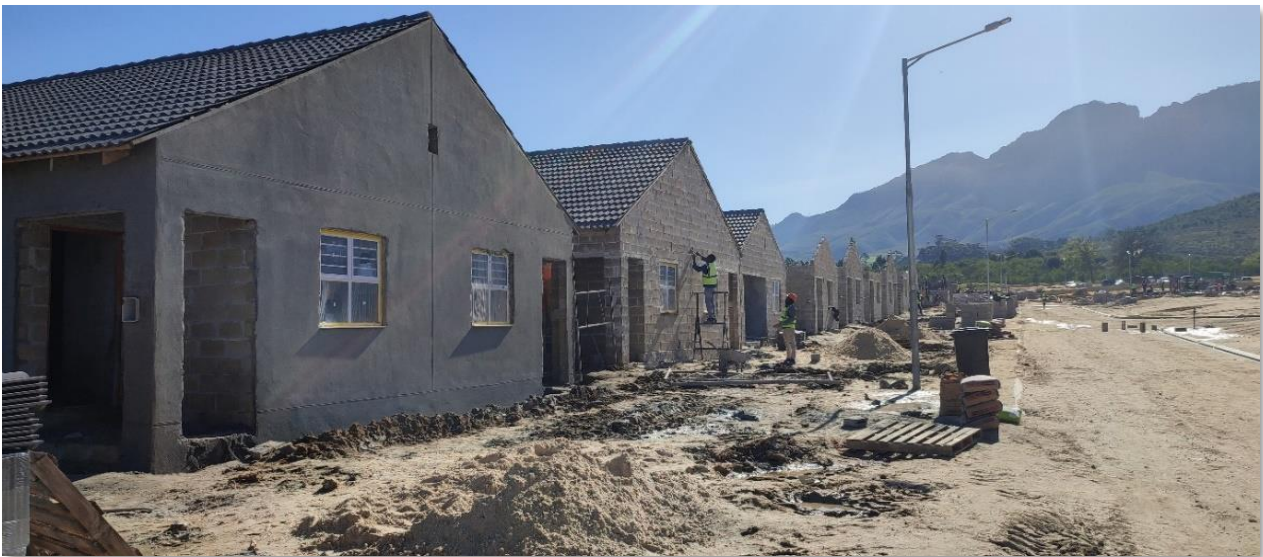
Figure 38: Ida's Valley Housing Development Project
