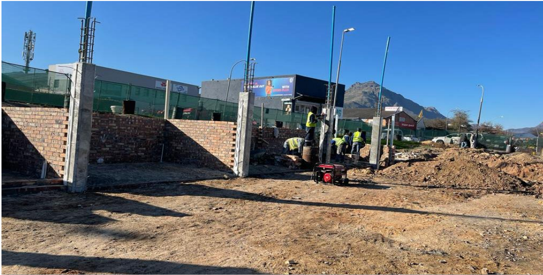
Figure 43: Construction of new taxi rank (Bird Street)
