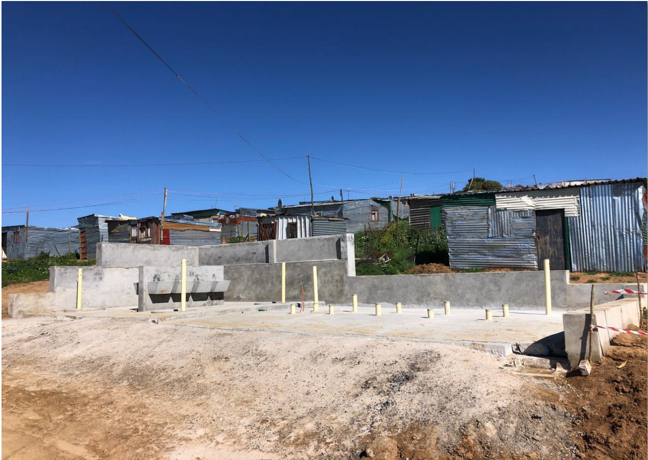
Figure 37: Construction of basic services, Watergang Informal Settlement
