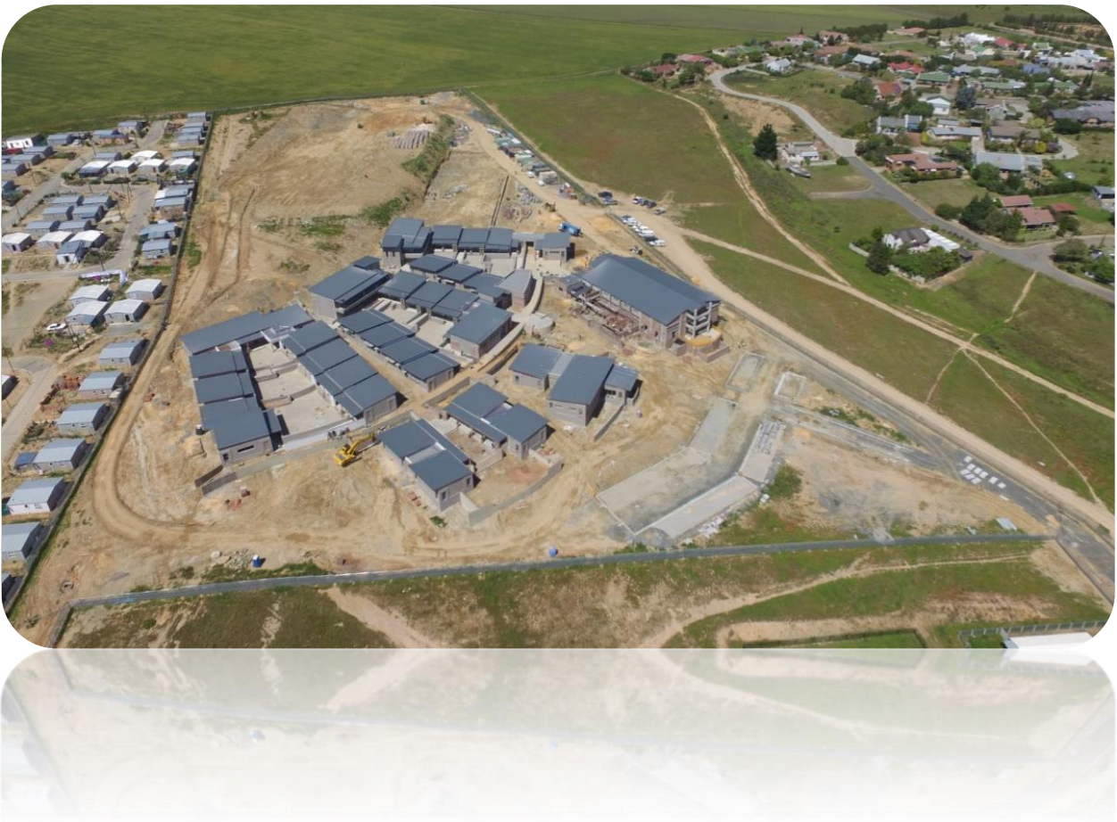
New School in Tulbagh
