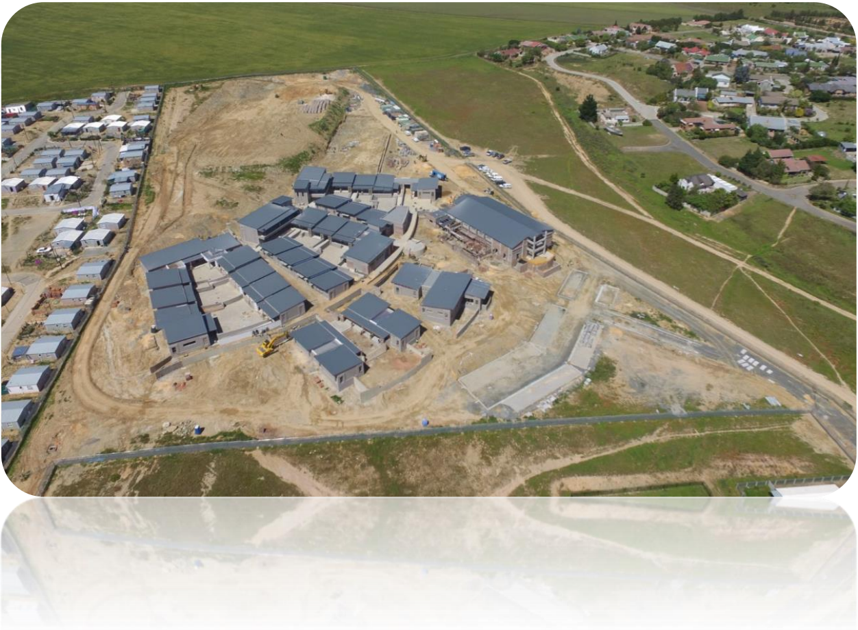
New School in Tulbagh
