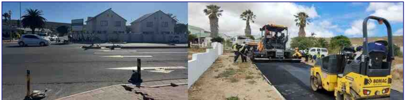
Intersection improvements at Saldanhaway & Doncaster intersection, Saldanha
