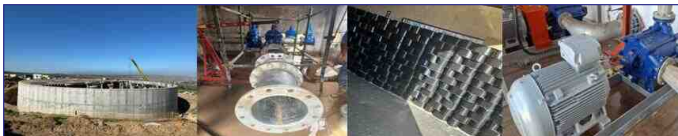
From L to R: Oliphantskop reservoir and bulk pipeline supply; Supply and delivery of smart water meters; Refurbishment of St Helena view bulk waterpump station
