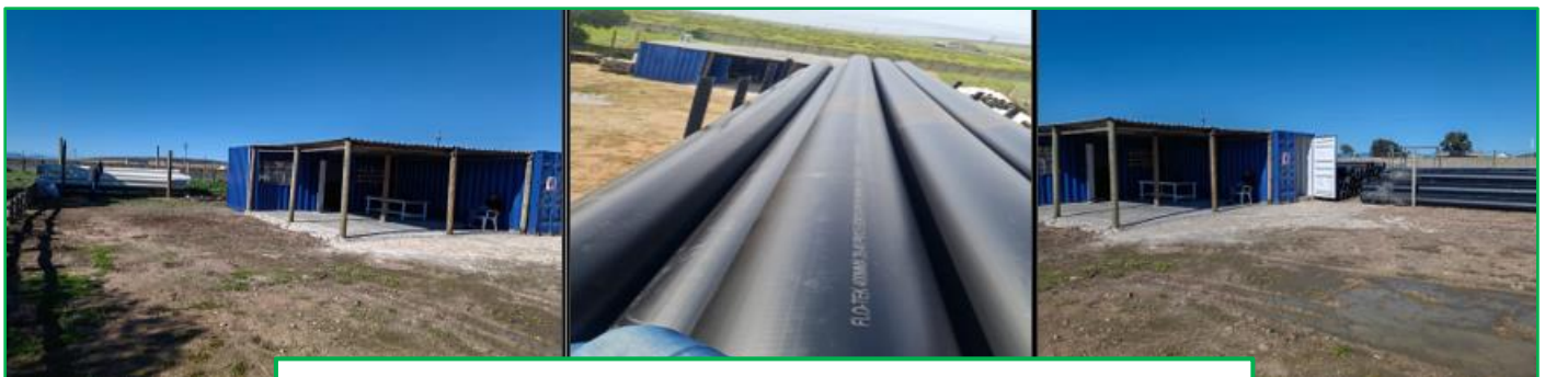
Bulk Sewer Infrastructure Upgrade Laingville Sewer Pumpstations & Pipelines Associated Works
