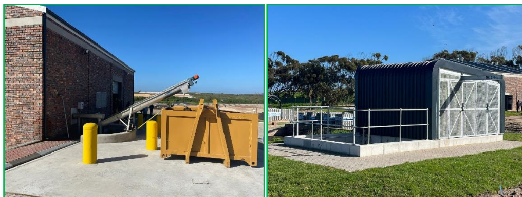
Langebaan Wastewater Treatment Works
