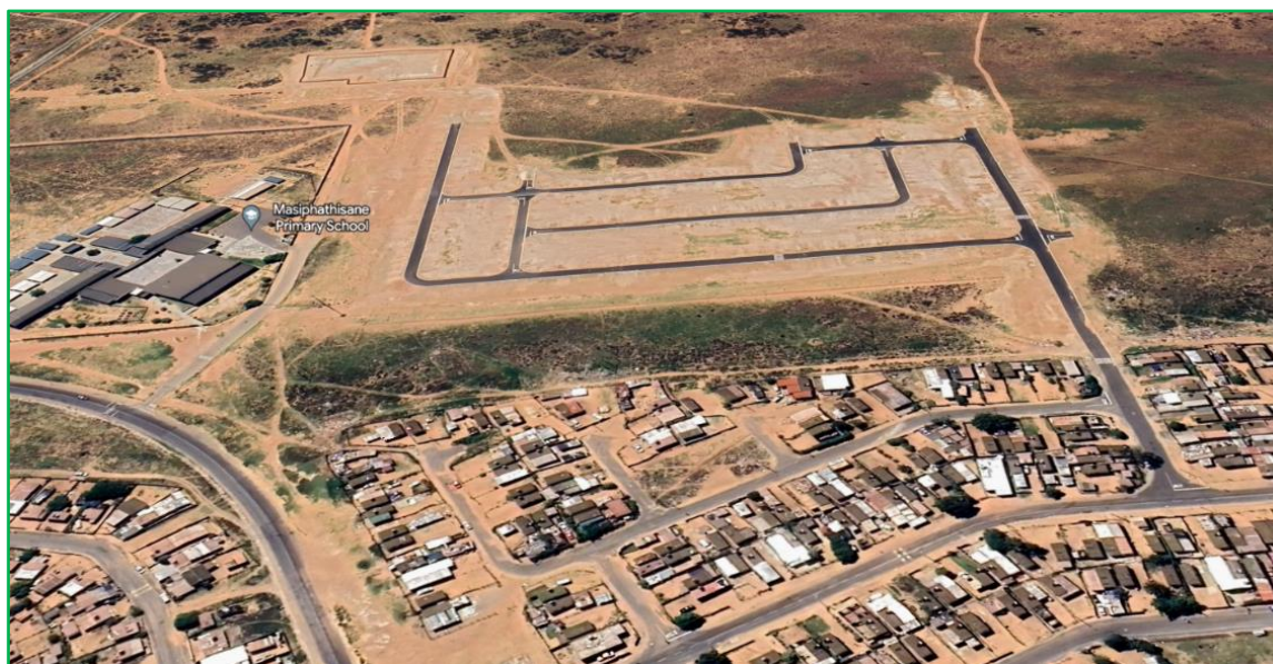
Witteklip 1155 : Phase 1 - Completed civil engineering services
