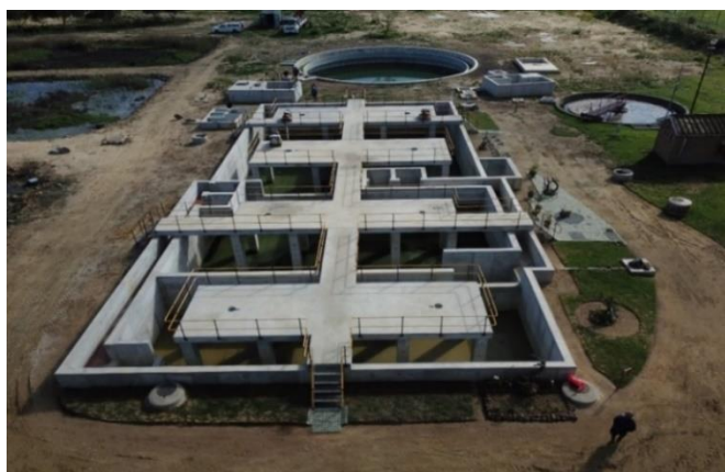
Upgrading of Porterville Sewerage Works
