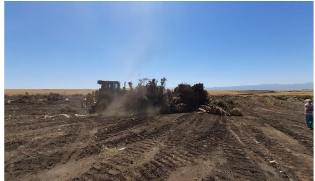
Photo of landfill site being cleared
