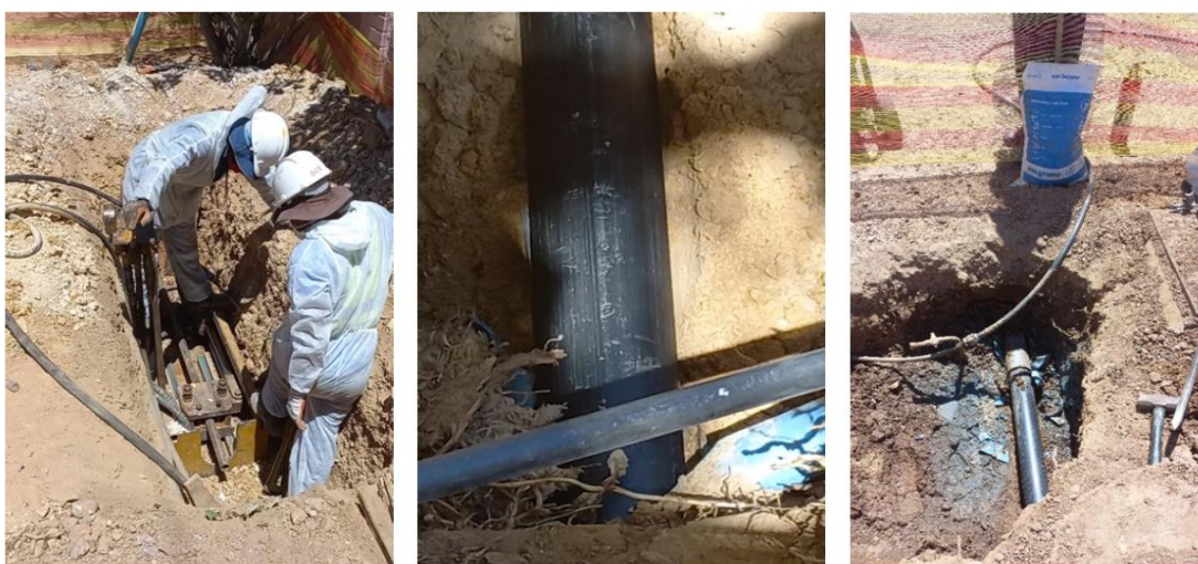
Pipe cracking
