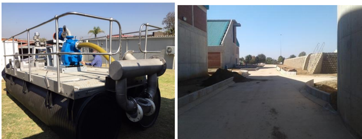
Figure 7: Completed Temba Purification Plant
