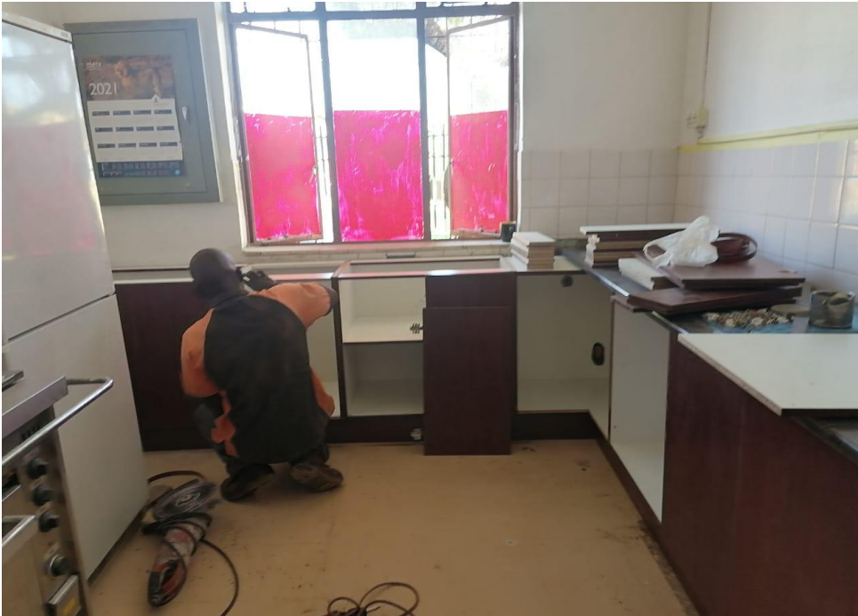
Figure 15: Maintenance work carried out at ECD centres
