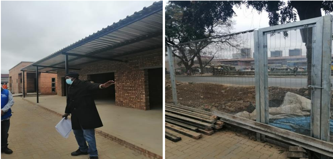
The completed Marabastad trading stalls
