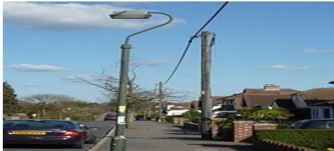
Figure 1: Example of an Insulated Bundle Electric Network
