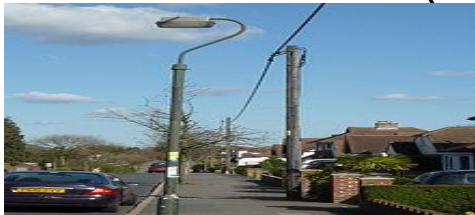
Figure 1: Example of an Insulated Bundle Electric Network
