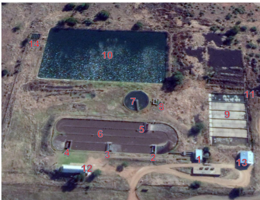
Fig 2 Existing Infrastructure Of The Warrenton WWTW
