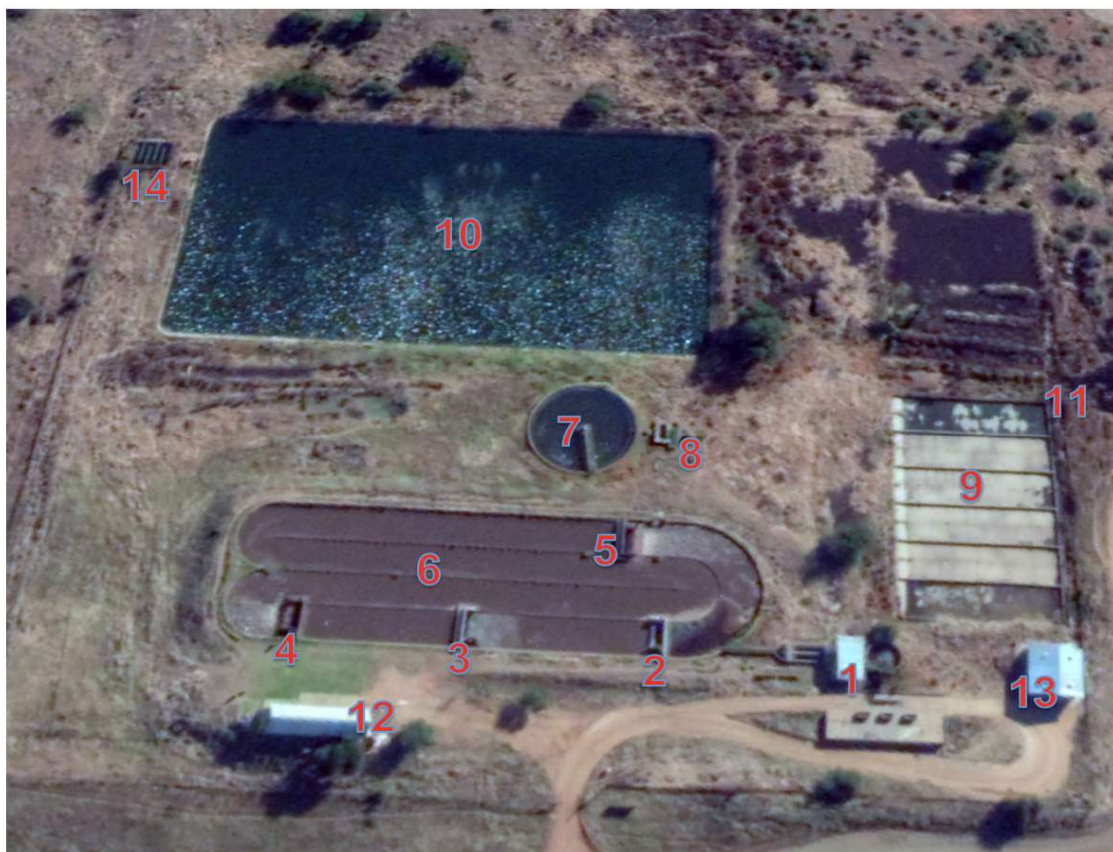
Fig 2 Existing Infrastructure Of The Warrenton WWTW
