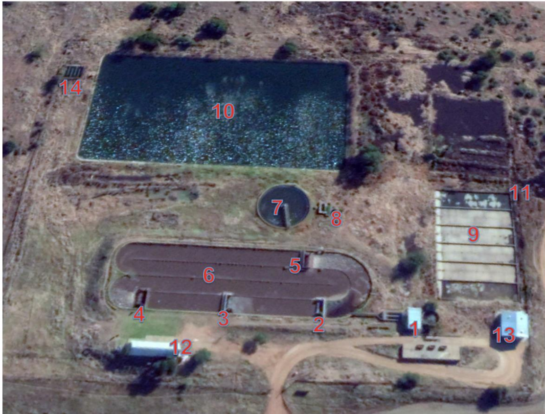
Fig 2 Existing Infrastructure Of The Warrenton WWTW
