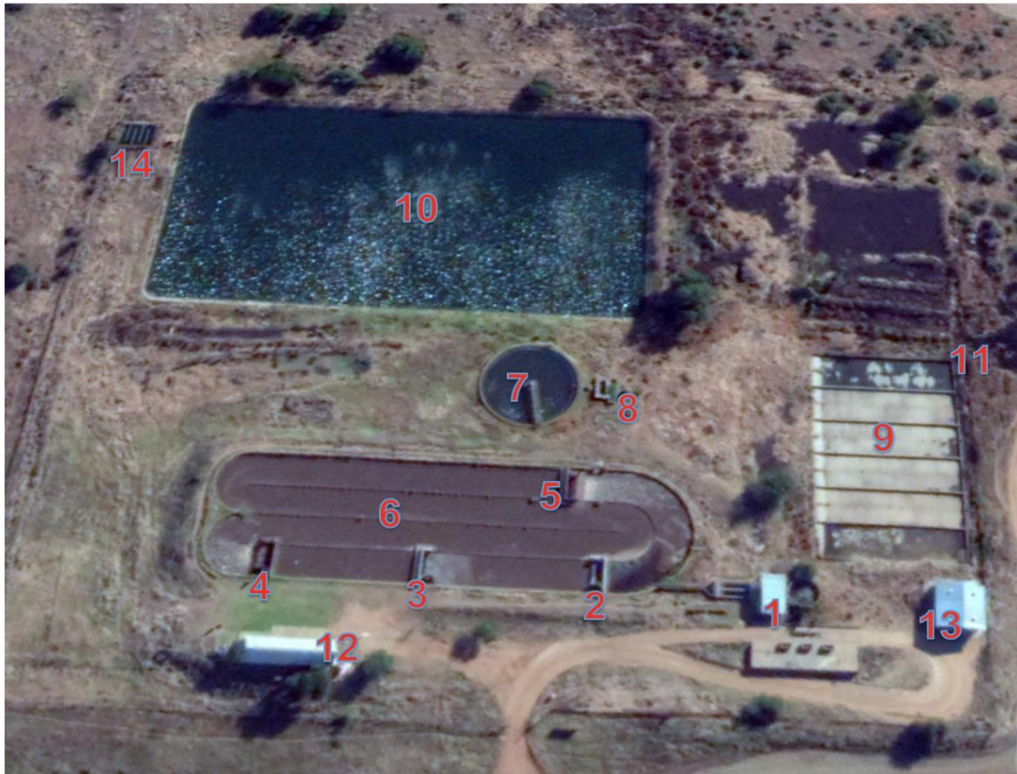
Fig 2 Existing Infrastructure Of The Warrenton WWTW
