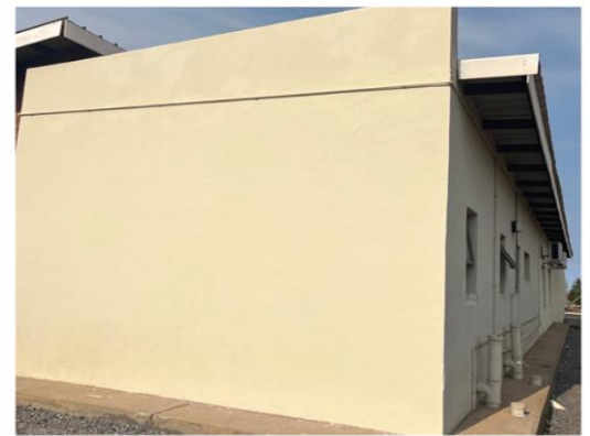
Photo.8 Newly painted Municipal Library Wall
