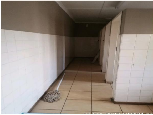
Photo3: Installation of tiles at Municipal Building.
