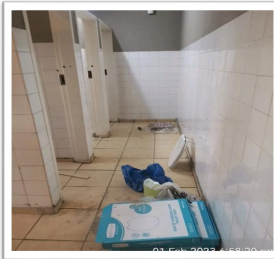
Photo1.: Replacement of toilet seats at Main Municipal Build
