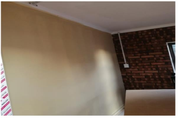
Photo5: Partitioning of Municipal Building
