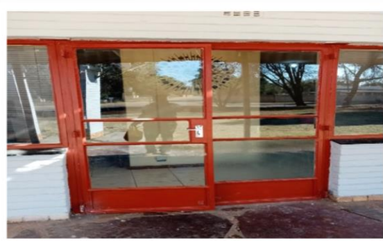
Photo.11 Newly painted glass door
