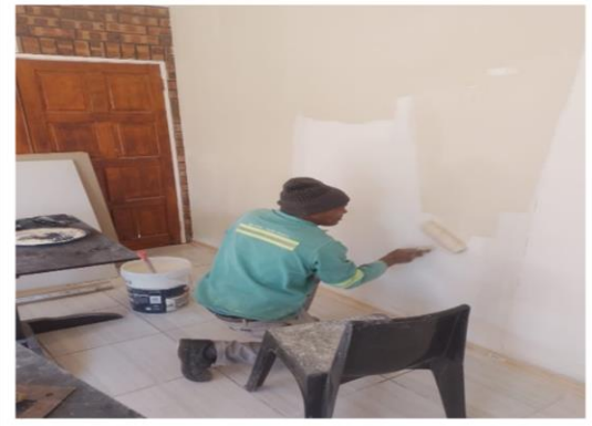
Photo6: Painting of partitioning board
