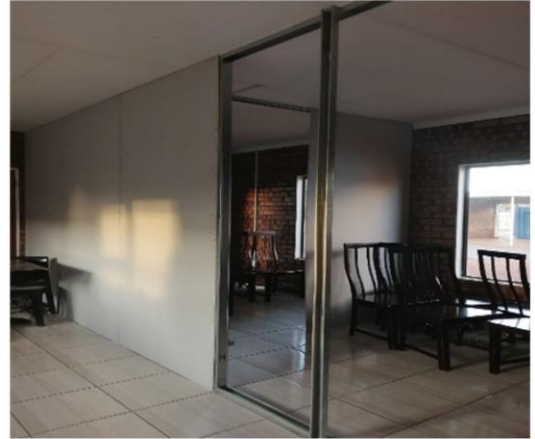
Photo4: Partitioning of Municipal Building
