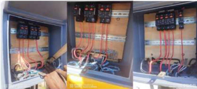
Wiring of Pole Boxes (Service connections)
