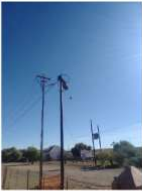
Installation of Pole Mounted Transformer
