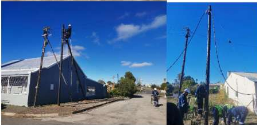
Stringing of ABC conductor
