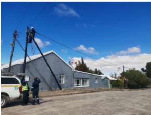
Wiring of Pole Boxes (Service connections)
