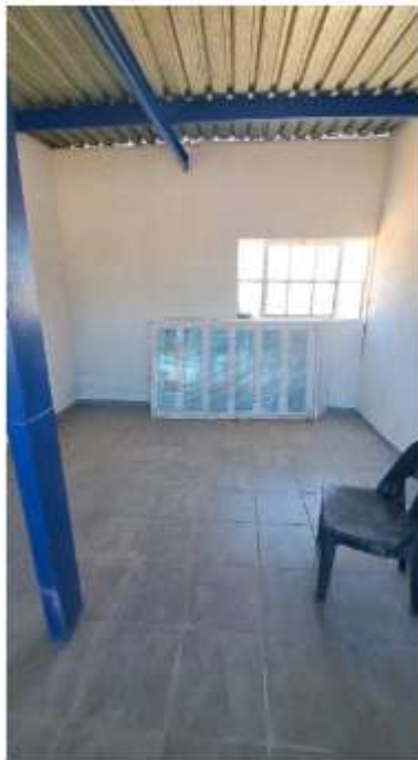
Finishing works in cloakroom
