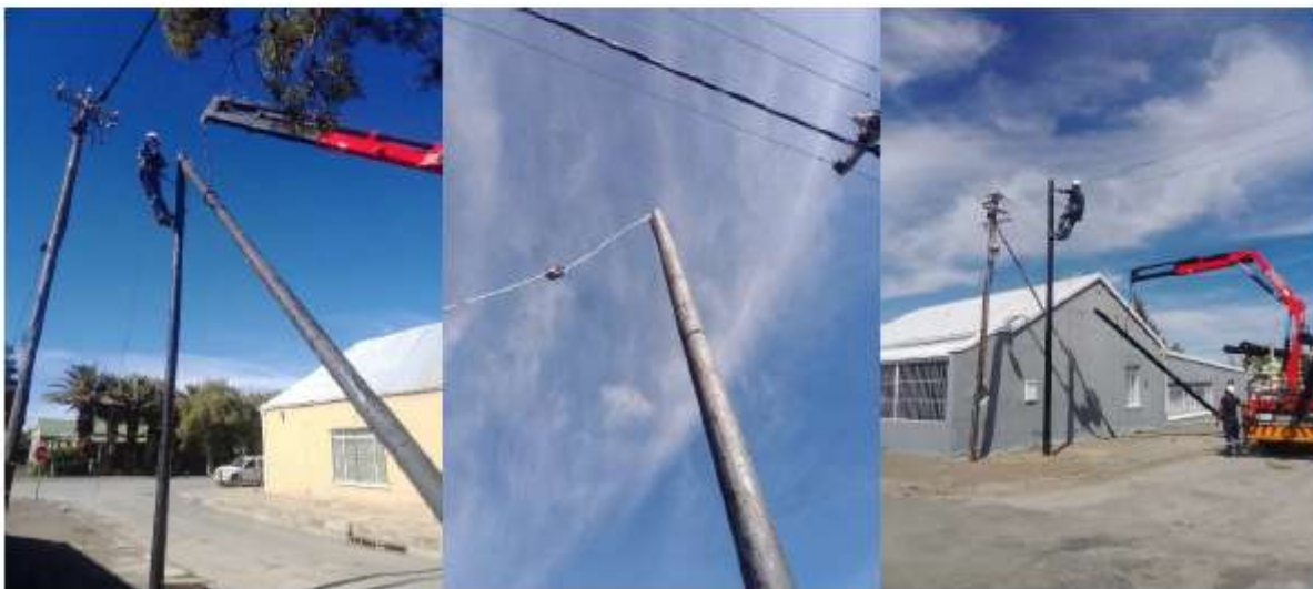
Line preparation: strut poles and stays
