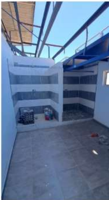
Finishing works in ablutions in cloakroom
