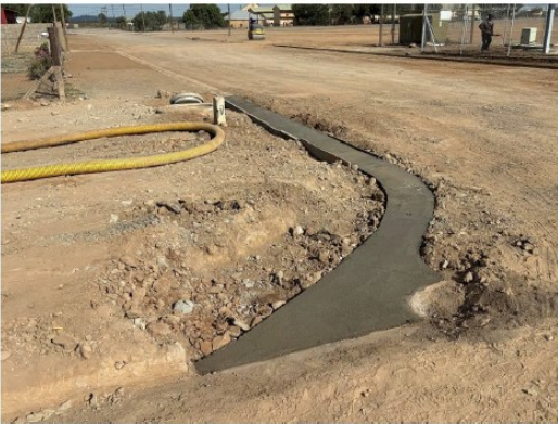
Reinstatement of kerbs and drainage gutters in Commercial Street
