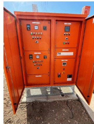
Motor Control Centre for the WW Pump Station
