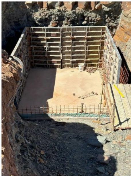
Completed excavation of pump station sump and concrete floor
