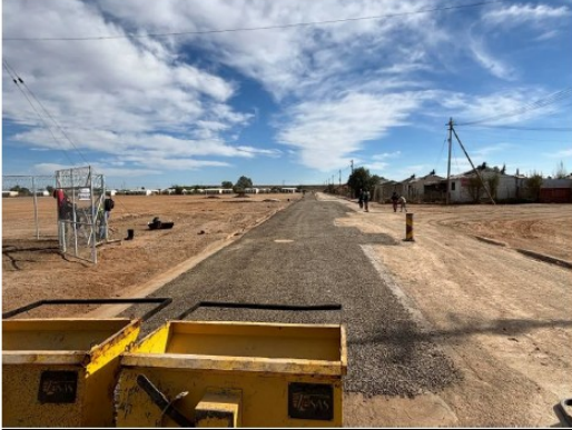
Completed repairs to Commercial Street road surface after sewer
