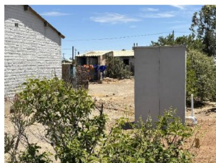
Fully assembled and connected pre-cast toilet structures
