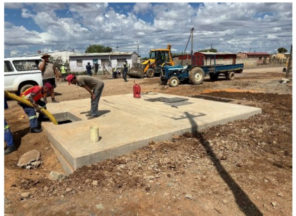
Completed Wastewater Sump for pump station
