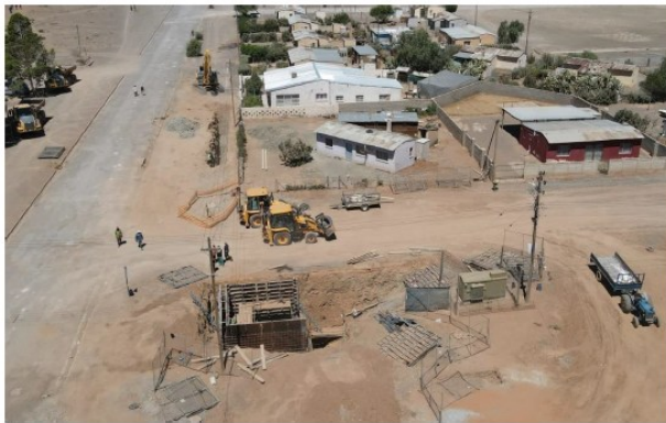
Construction of Wastewater Pump Station sump cnr of Prins and Commercial Streets, Fraserburg
