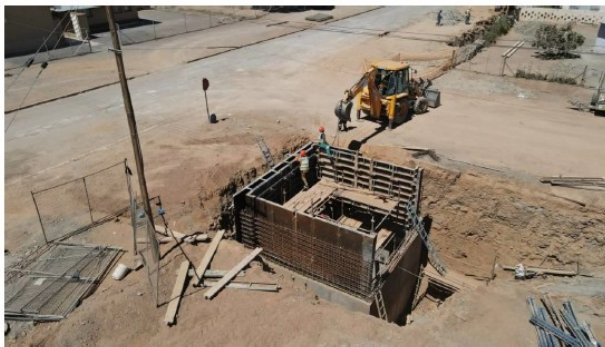
Erection of shutters for casting of pump station sump walls
