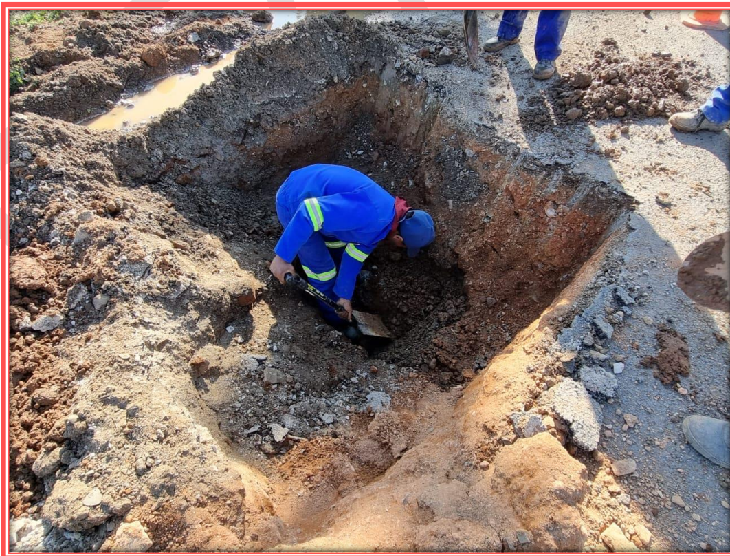
Pictures 1: Trench digging
