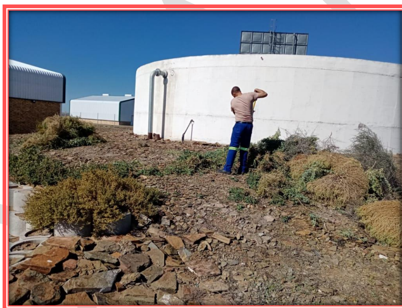
Pictures 4: Waternetwork cleaning - Brandvlei
