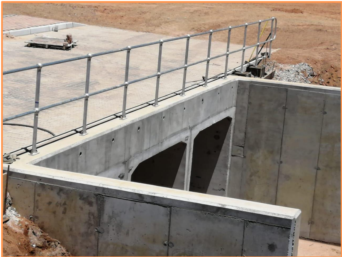
Pictures 4: The bridge and stormwater channels
