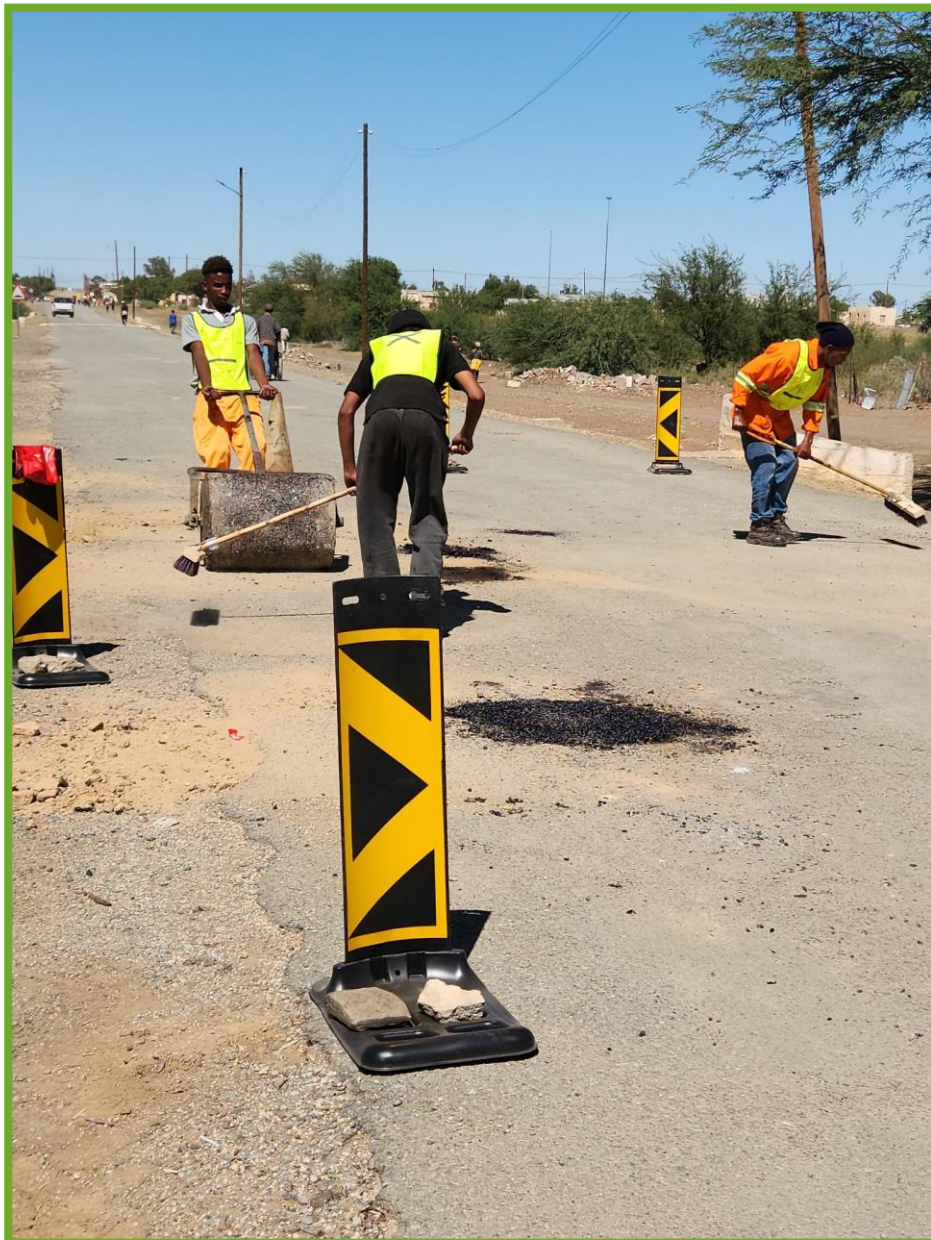
Pictures 6: Closing of potholes
