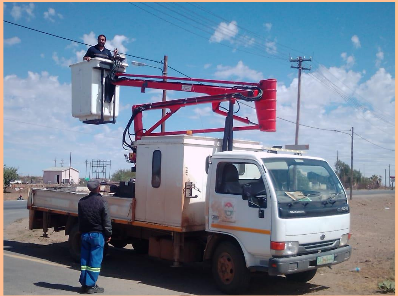
Pictures 5: Electrical team hard at work
