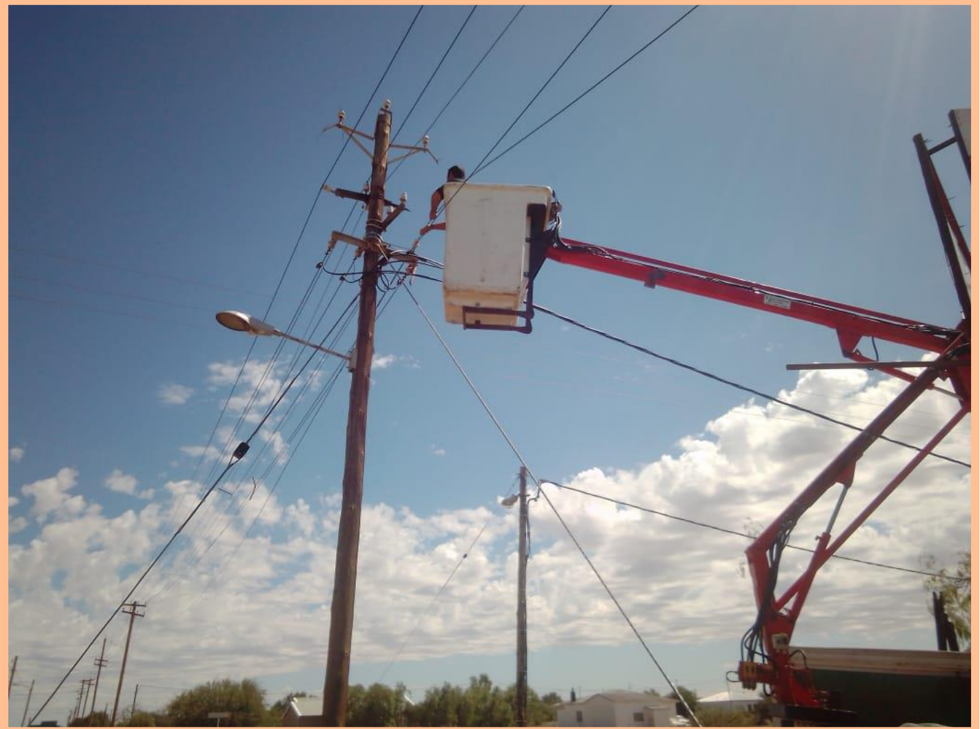
Pictures 6: Restoring electrical connections
