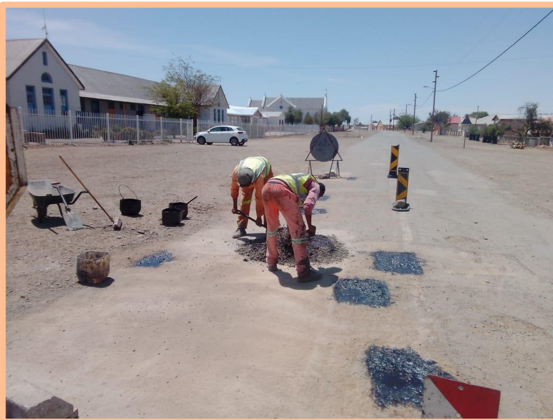
Pictures 1: Fixing potholes
