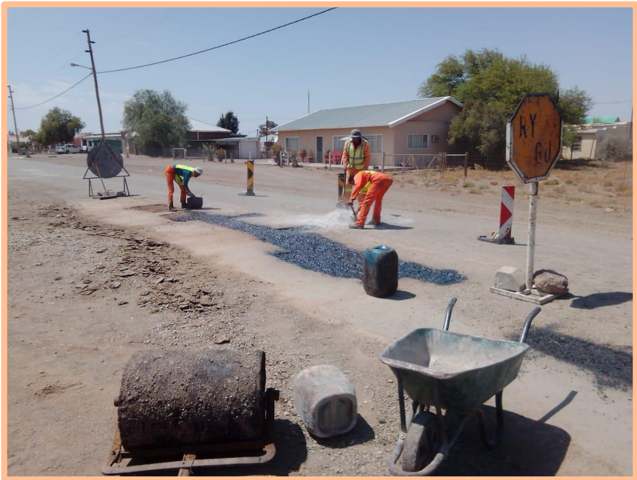
Pictures 9: Fixing potholes
