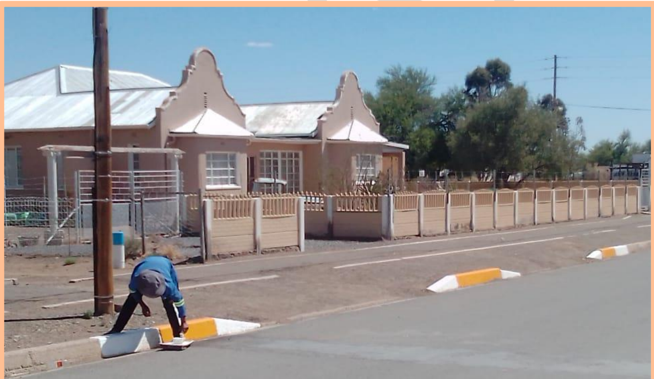
Pictures 12: Painting of roadmarkings
