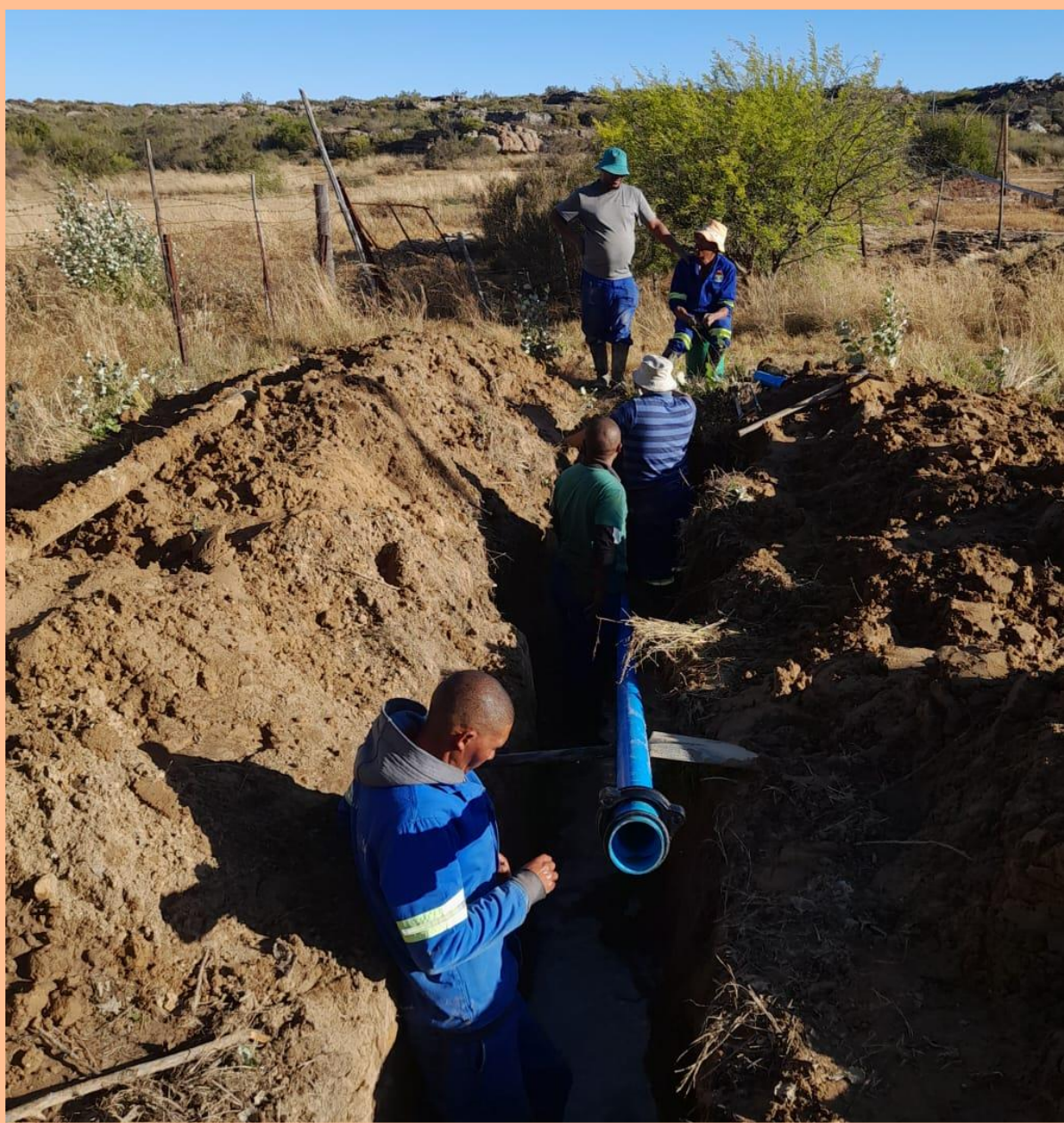
Pictures 4: Replacement of water pipe
