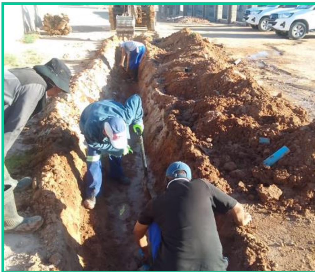
Picture 12: Routine Maintenance
