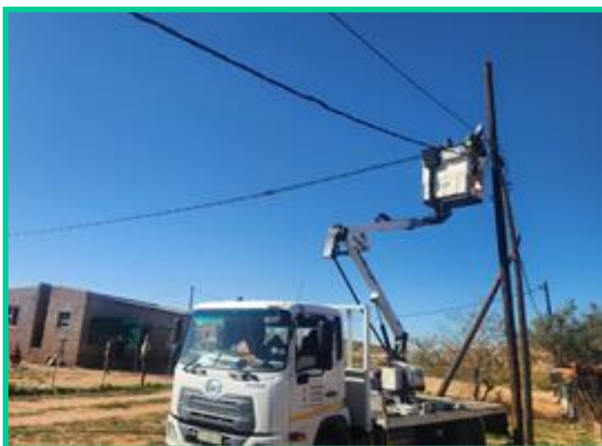
Picture 18: Routine Maintenance
