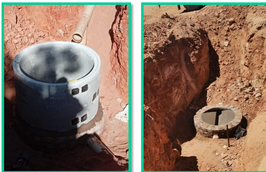
Picture 16: Okiep Sewer - Rocky Ridge project
