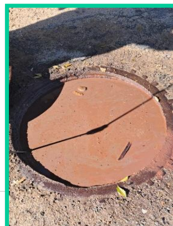
Picture 15: Routine Maintenance works
