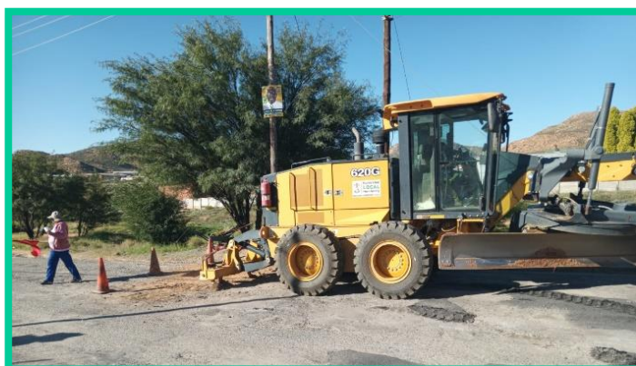
Picture 25: Upgrade of Waterkant Skool Street intersection
