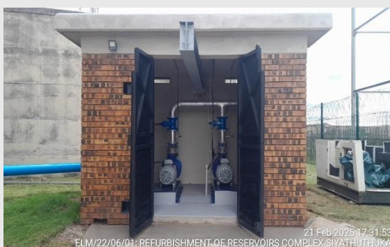
Figure 5&6: Pump house, mechanical and electrical components
