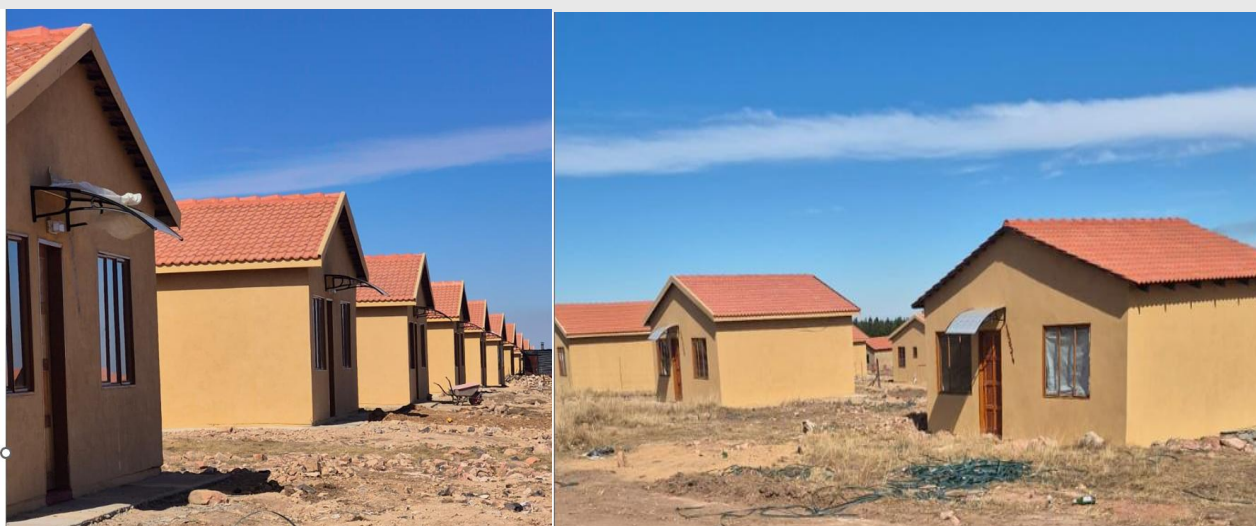
Figure 19&20: Newly constructed low-cost housing
