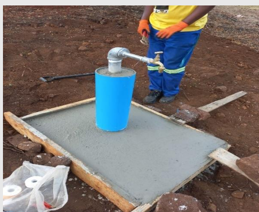
Figure 5&6: Standpipes installed
