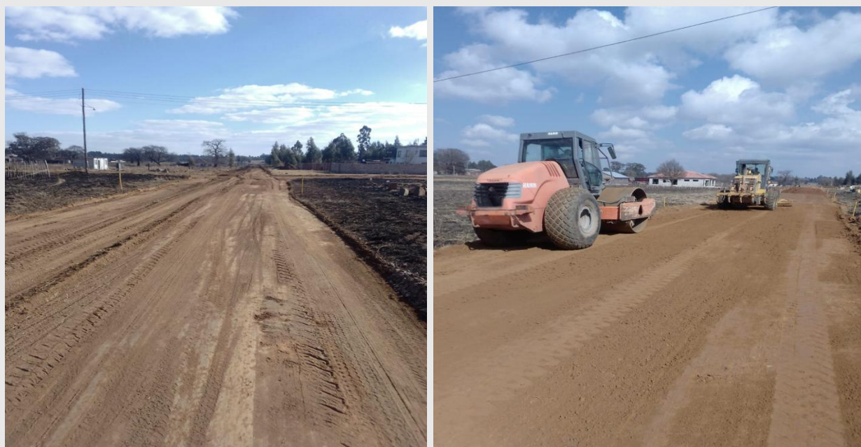
Figure 23&24: regravelling
