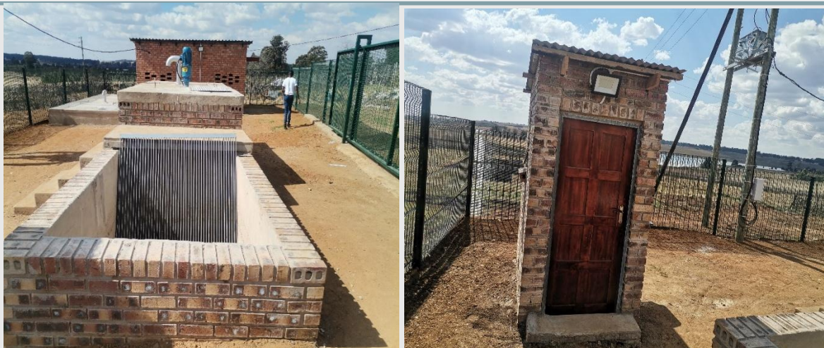
Figure 11&12: Civil and Building works
