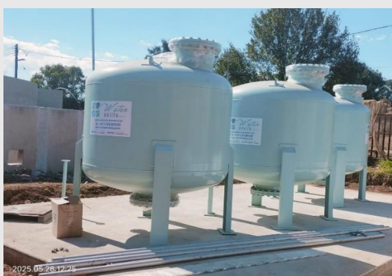
Figure 3&4: Pressure filters & recycled water pond
