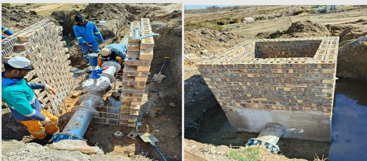
Figure 13&14: Installation of valve and valve chamber
