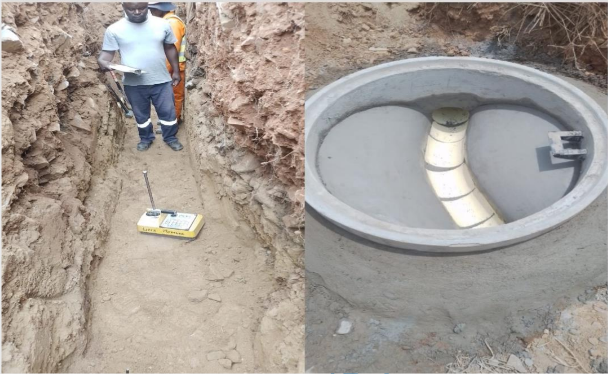
Benching and Compaction testing at Emthonjeni sewer outfall
