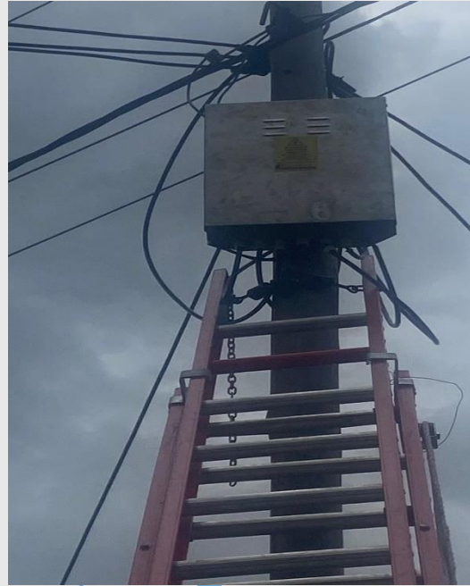
Figure 5: Installation of kiosks and pole top box at Watervaal Boven and Emgwenya
