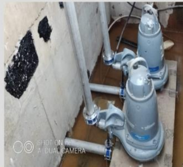
Photo 5: Pumps Installed at Madala Pump station
