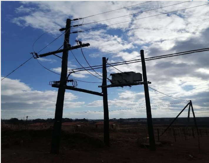
Figure 3: Construction of MV infrastructure including 200kVa pole transformer
