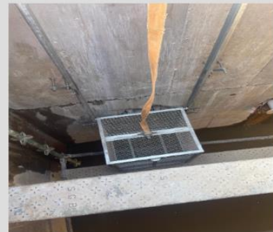
Photo 6: Screen Basket installed in Madala Pump station
