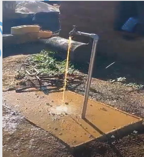
Figure 3: Standpipe installed
