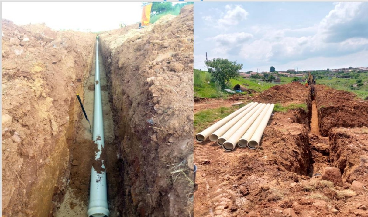
Pipe laying at Emthonjeni sewer outfall
