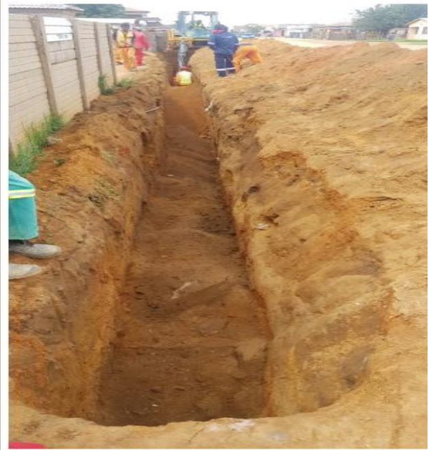
Fig 2: Partially backfilled trench for compaction
