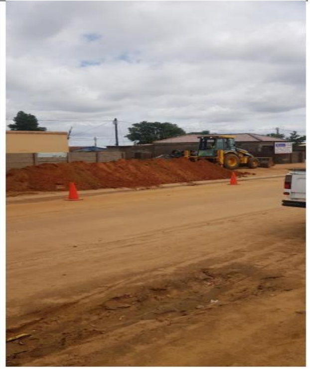
Fig 4: Excavation of MHD line
