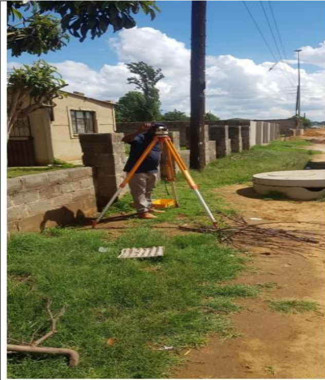
Fig 3: Surveyor giving levels on the trench
