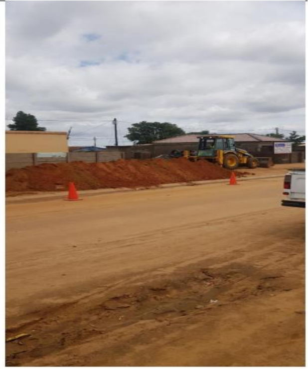
Fig 4: Excavation of MHD line
