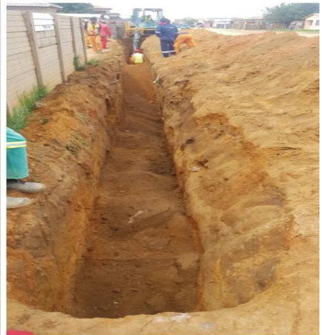
Fig 2: Partially backfilled trench for compaction
