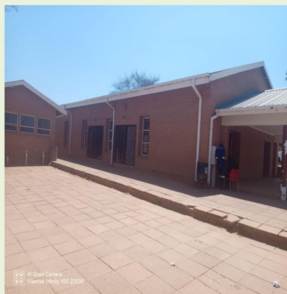
FIGURE: 4 JINNAH PARK COMMUNITY HALL
