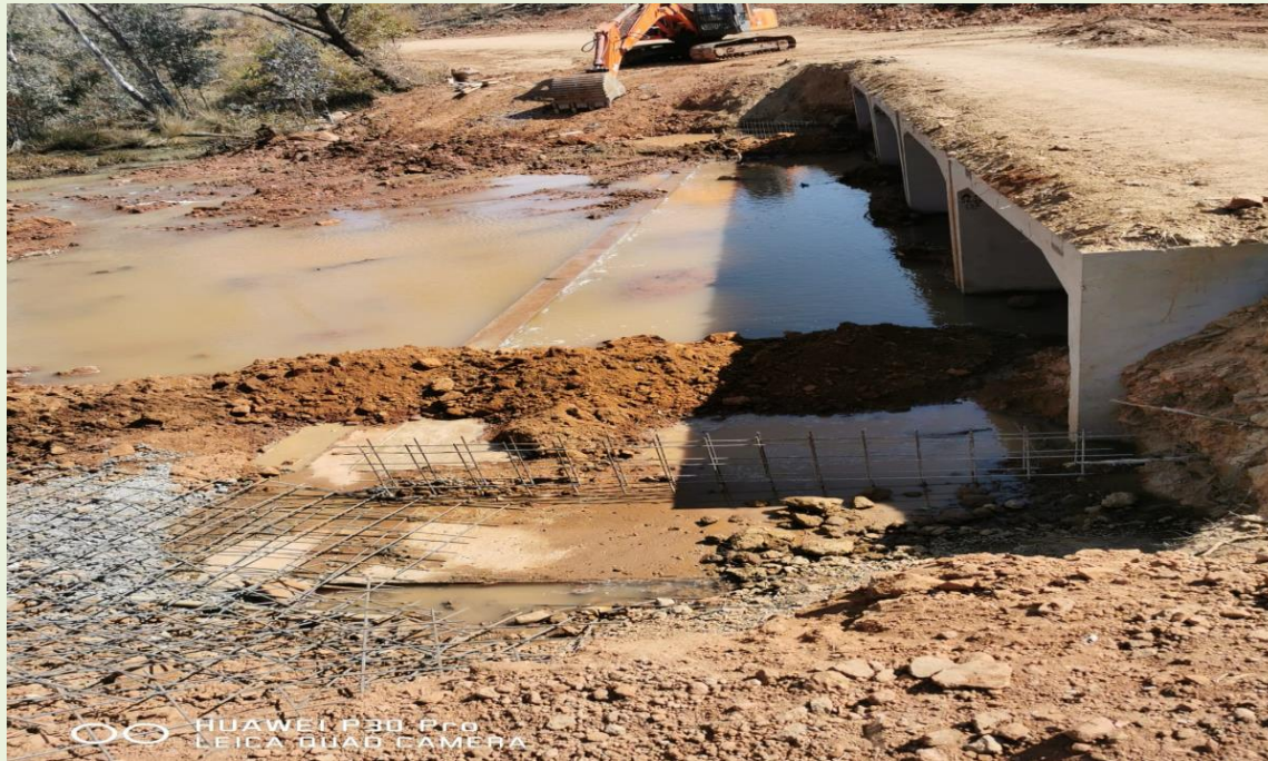
IMAGE 1: REHABILITATION OF ACCESS ROAD TO THE WARMBAD DAM
