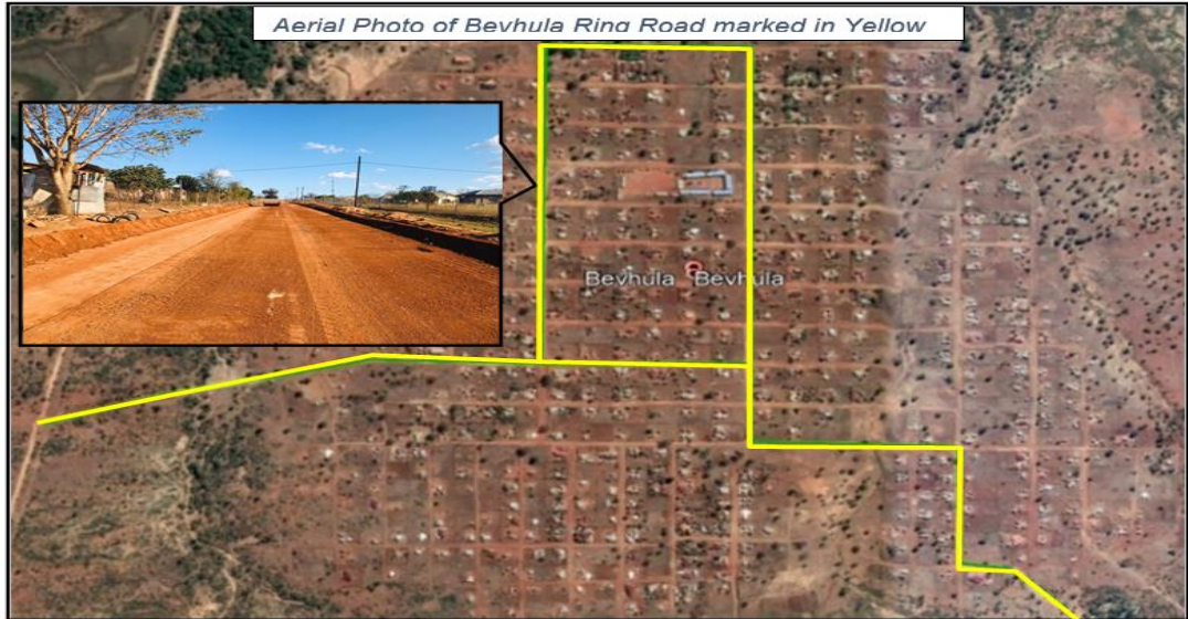
Picture 8 Upgrading of Bevhula Ring Road.
