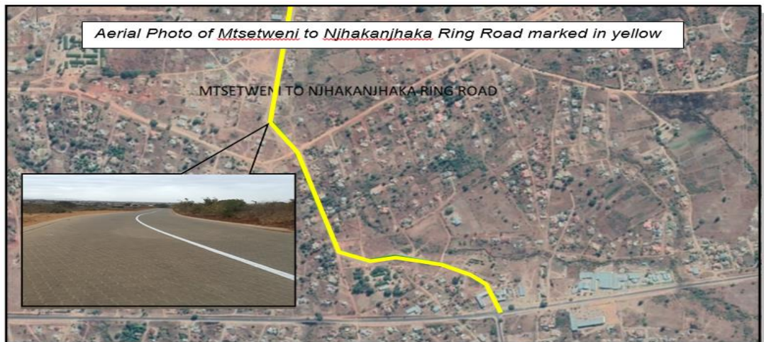
Upgrading of Mtsetweni to Njhakanjhaka Ring Road Phase 2
