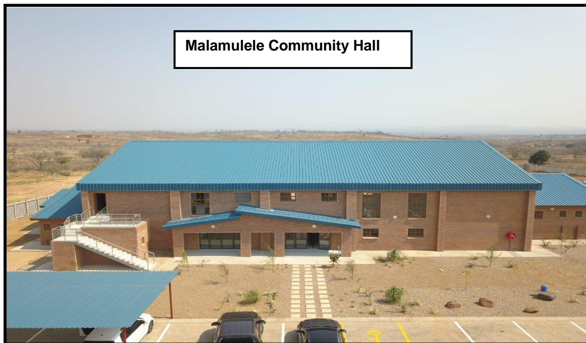
Construction of Malamulele Community Hall
