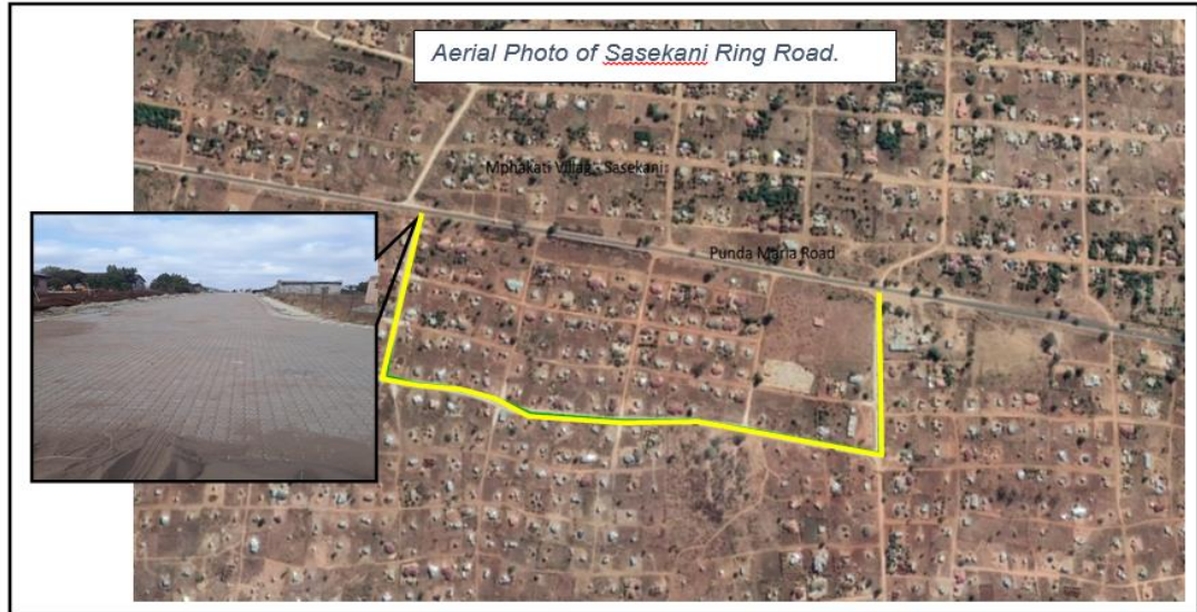
Upgrading of Sasekani Ring Road
