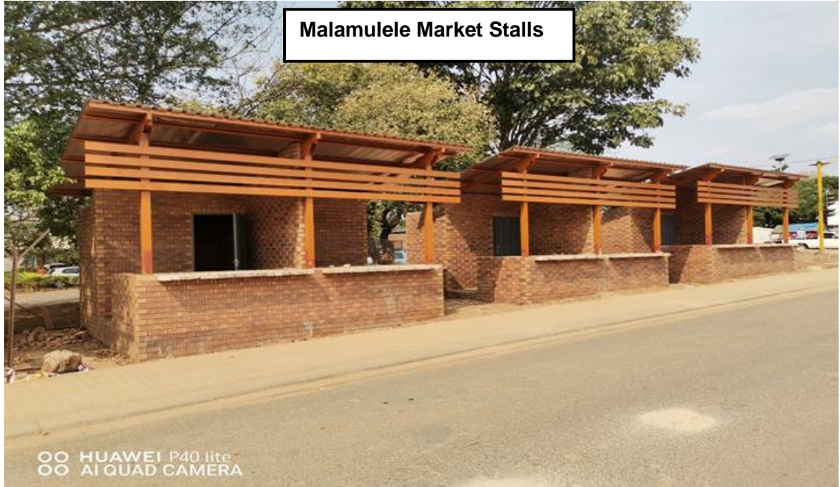
Construction of Malamulele Market Stalls
