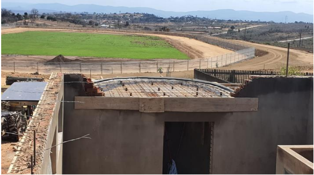
Picture 12 Upgrading of Malamulele Stadium
