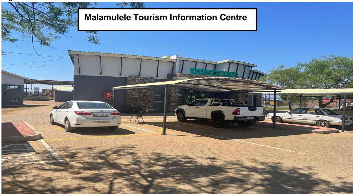
Construction of Malamulele Tourism Information Centre
