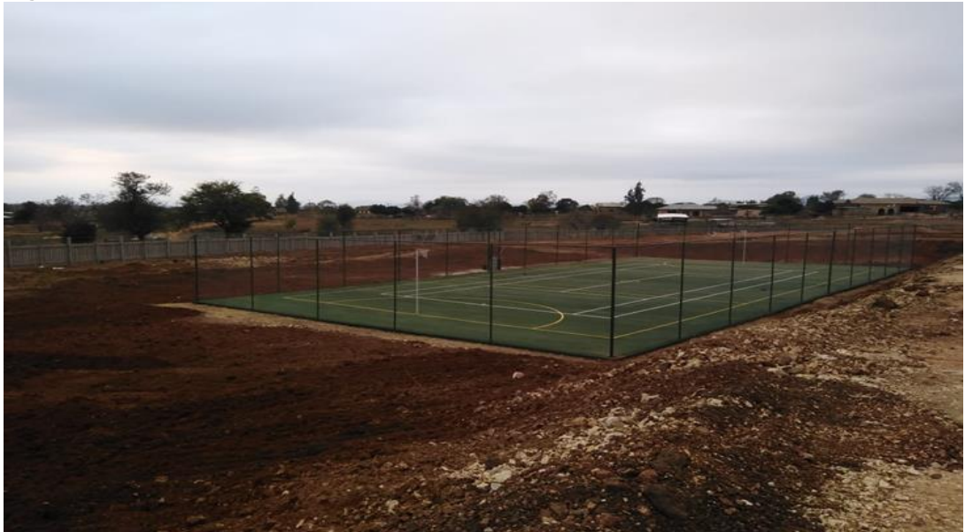
Picture 13 Construction of Davhana Stadium Phase 1
