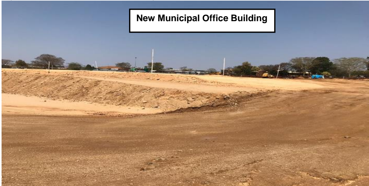
Construction of New Municipal Office Building
