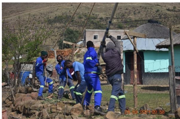
Installation of lightning conductors
