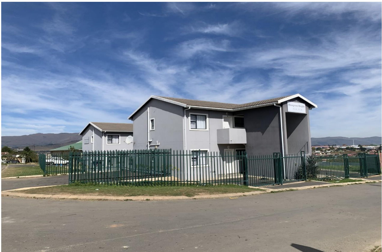
Bhongweni Heights 133 Units in progress
