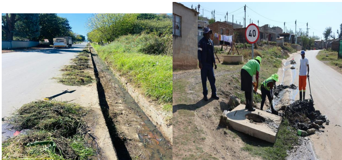
STORM WATER DRAIN CLEANING
