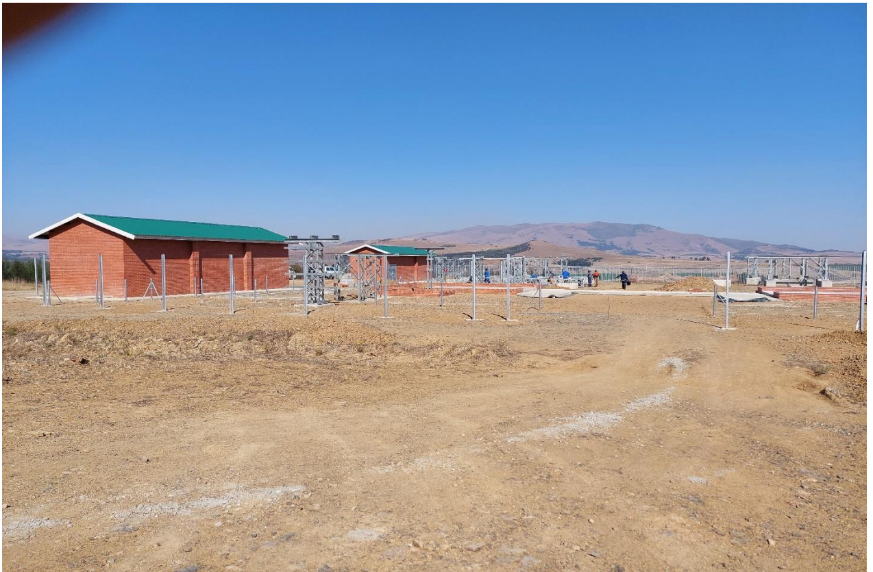
SINGISI SUBSTATION PROJECT
