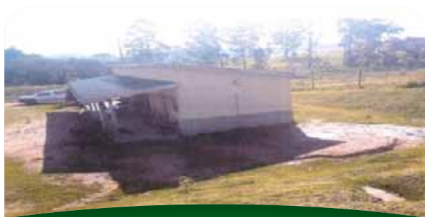
Refurbishment of change rooms in Vlakspruit cemetery – before refurbishment
