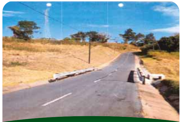
Vlakspruit cemetery Access road: after rehabilitation
