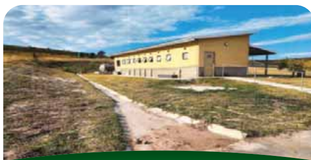
Refurbishment of change rooms in Vlakspruit cemetery – after refurbishment
