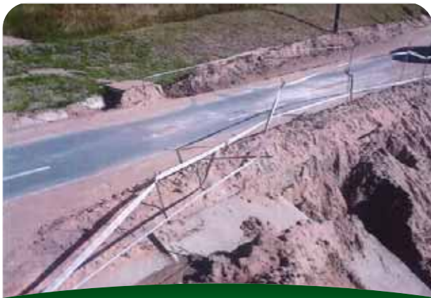
Vlakspruit cemetery Access road: before rehabilitation
