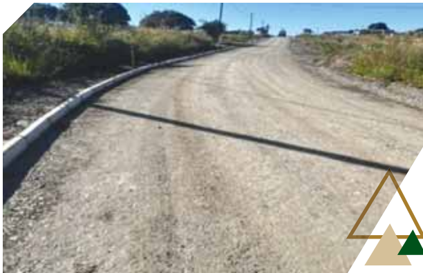
WATER WORKS ROADS PHASE 2 (WARD 26) - Construction in progress
