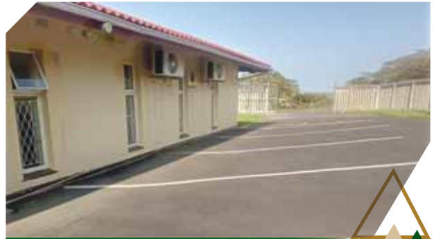
Resurfaced parking area
