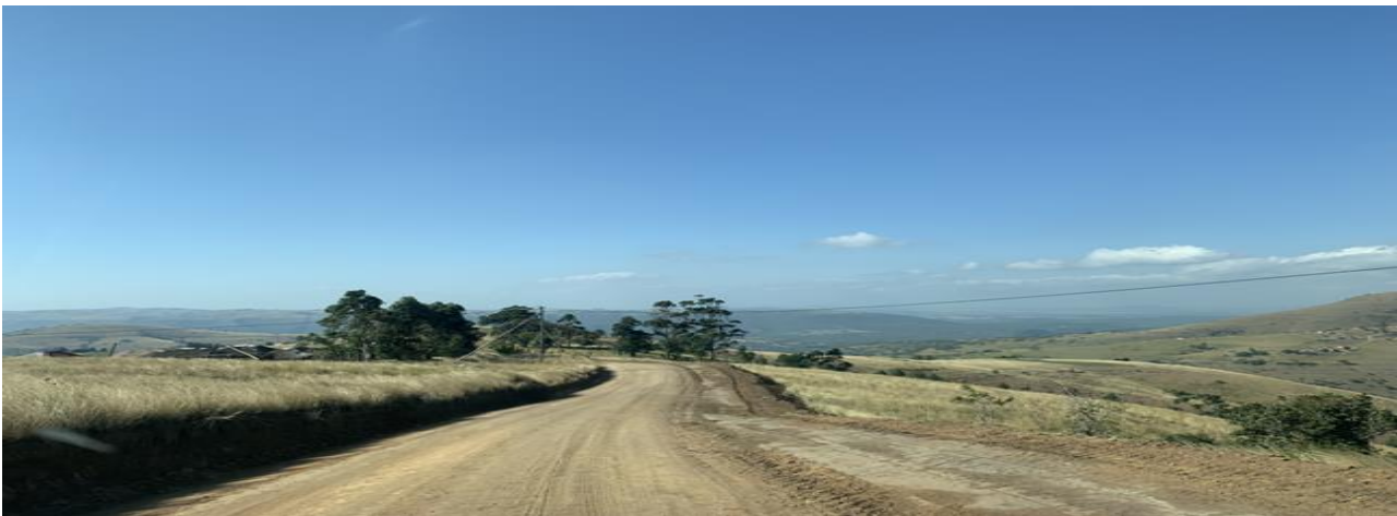
Image 3 – Ndundulu Gravel Road in Ward 8 ( R 6,200,403.00)
