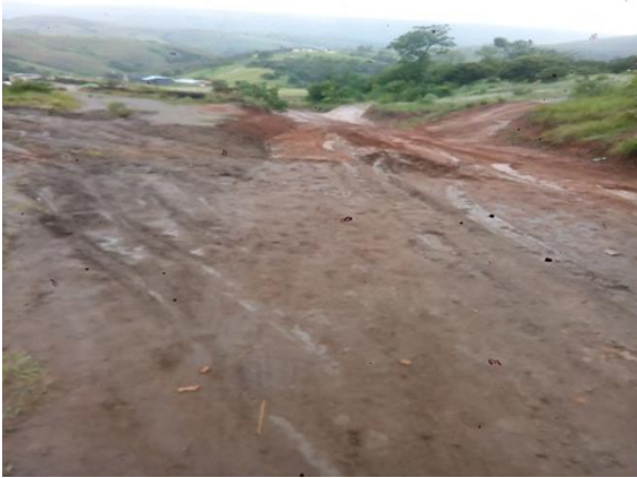
Image 22 - Blading and opening of residential roads in ward 9
