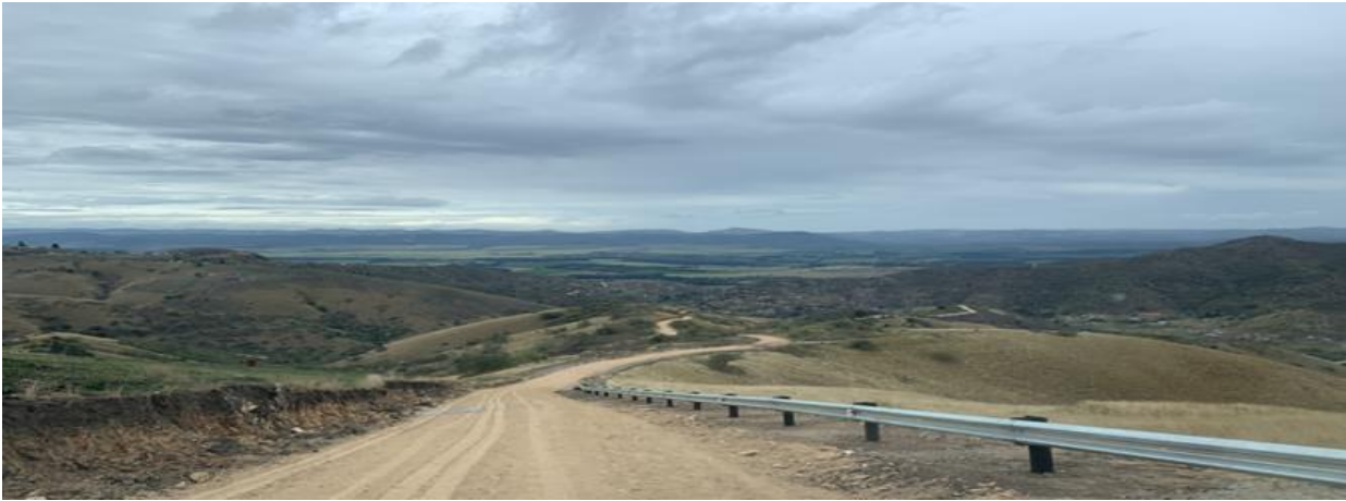
Image 4 - Makhubalo Gravel Road in Ward 9 – R 3,501,542.31
