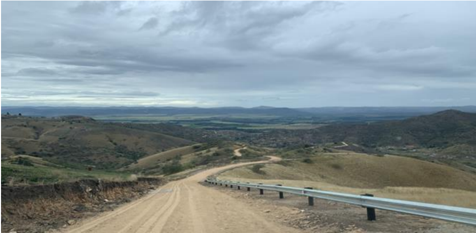
Image 24 - Makhubalo Gravel Road in Ward 9 – R 3,501,542.31
