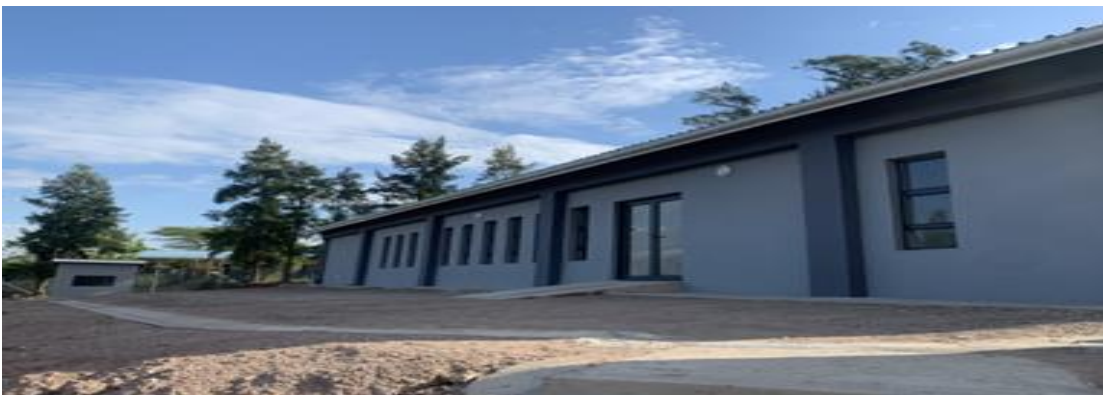
Image 8 - Bedlane Community Hall in Ward 8 – (R 5,113,428.70)
