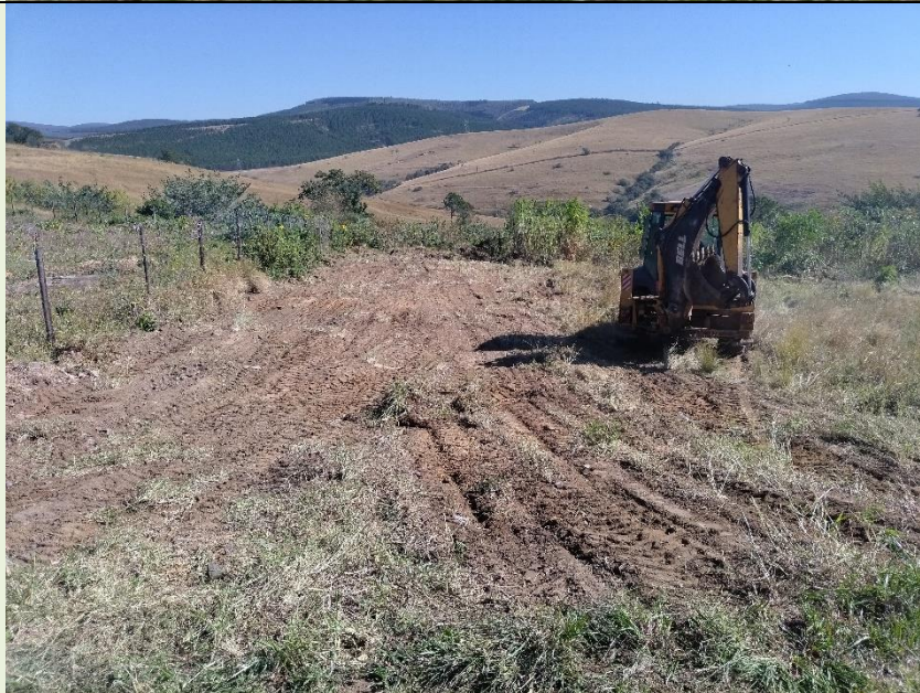
Road verge clearing in High Street.
