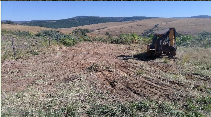
Road verge clearing in High Street.
