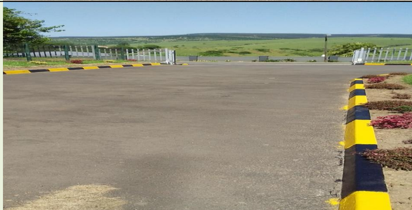
Protection services parking after road marking.
