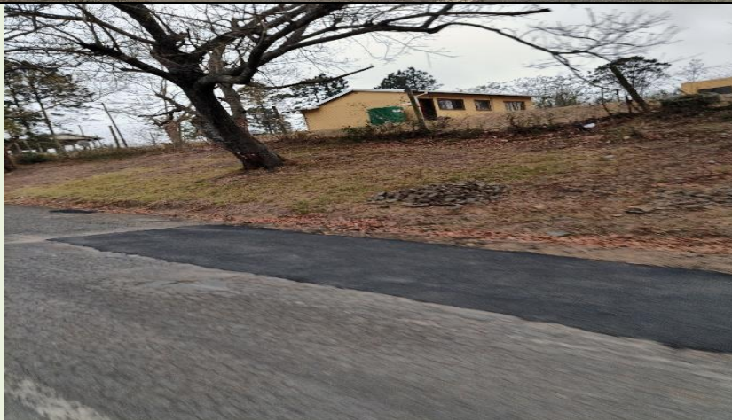
Patching and compaction of urban roads Melmoth Town.
