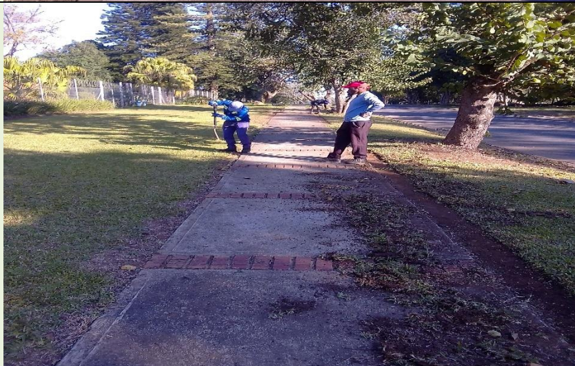
Trimming and cleaning of pedestrian pathway in Hammer Street.
