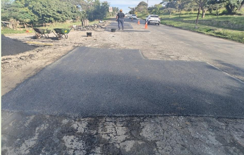
Priming and Patching of Piet Retief Roads in Melmoth Town.
