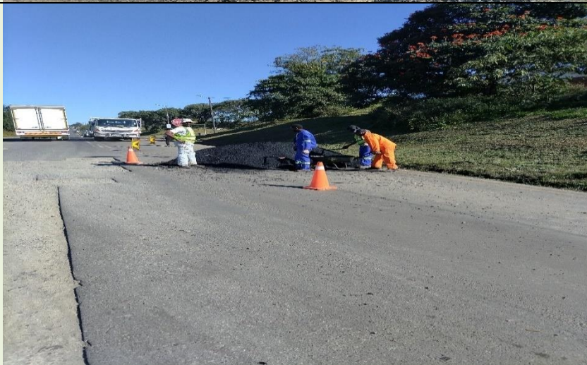
Priming and Patching of Piet Retief Roads in Melmoth Town.
