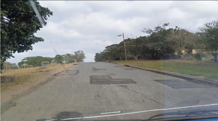
Patching and compaction of urban roads Melmoth Town.
