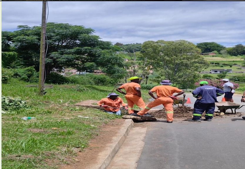
Unblocking and cleaning of storm-water drain in Melmoth Town.
