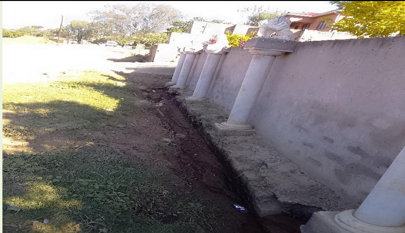
Unblocking of open drains in Thubalethu Township in Melmoth Town .
