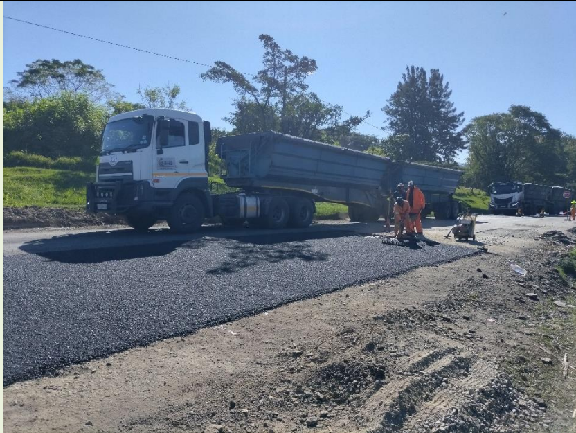
Priming and Patching of Piet Retief Roads in Melmoth Town.
