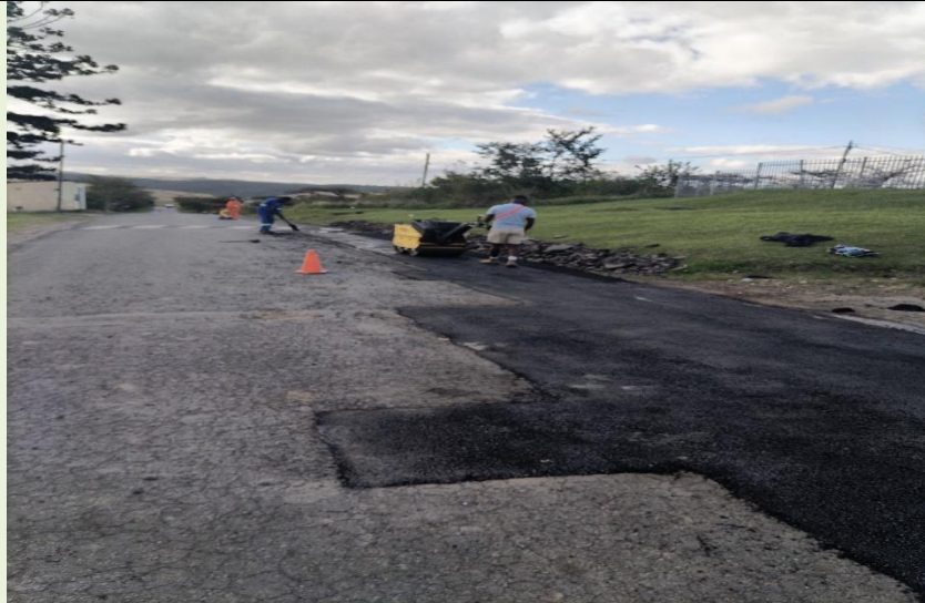
Patching and compaction of urban roads Melmoth Town.
