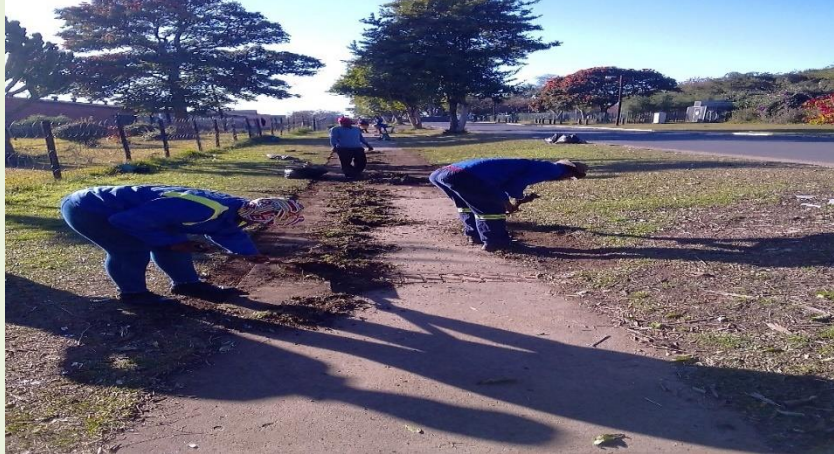
Trimming and cleaning of pedestrian pathway in Hammer Street.
