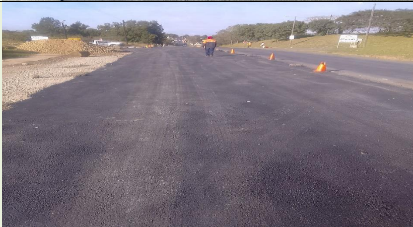
Priming and Patching of Piet Retief Roads in Melmoth Town.
