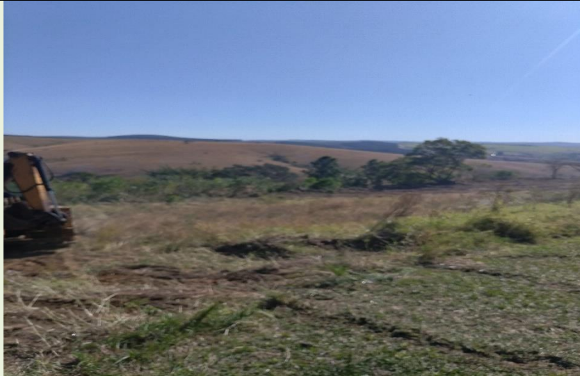
Road verge clearing in High Street.
