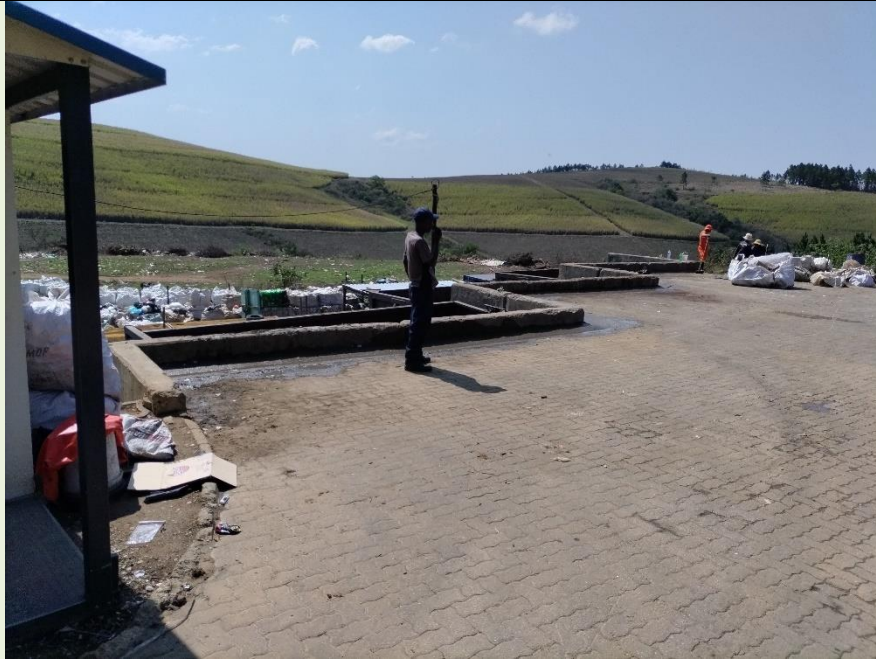
The municipal transfer station clean platform.
