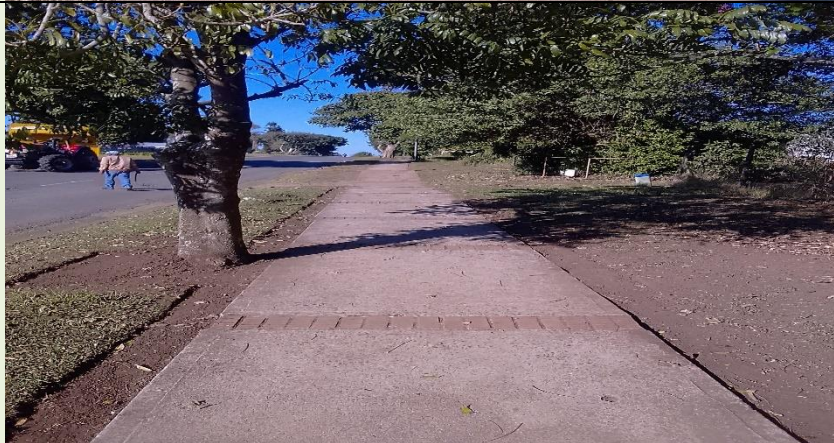
Trimming and cleaning of pedestrian pathway in Symmonds Street.
