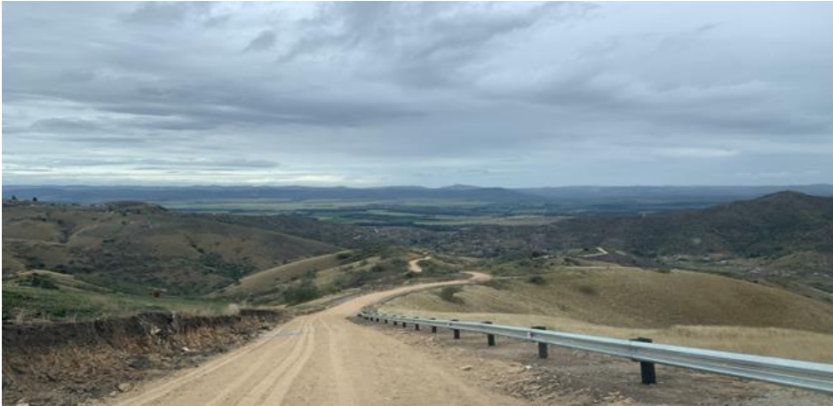
Image 25 - Makhubalo Gravel Road in Ward 9 – R 3,501,542.31
