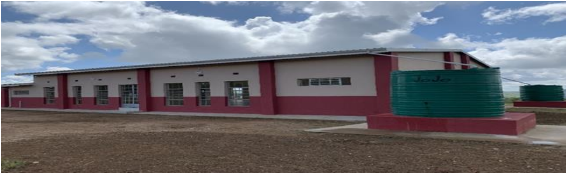
Image 2 -Njomelwano Community Hall in Ward 3
