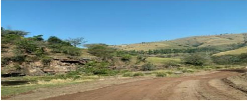
Image 10 - Ofankomo Gravel Road in Ward 3 – (R 4,971,24.06)
