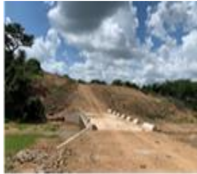
Image 5 - Ntilingwane Gravel Road in Ward 12 – R 4,845,180.00
