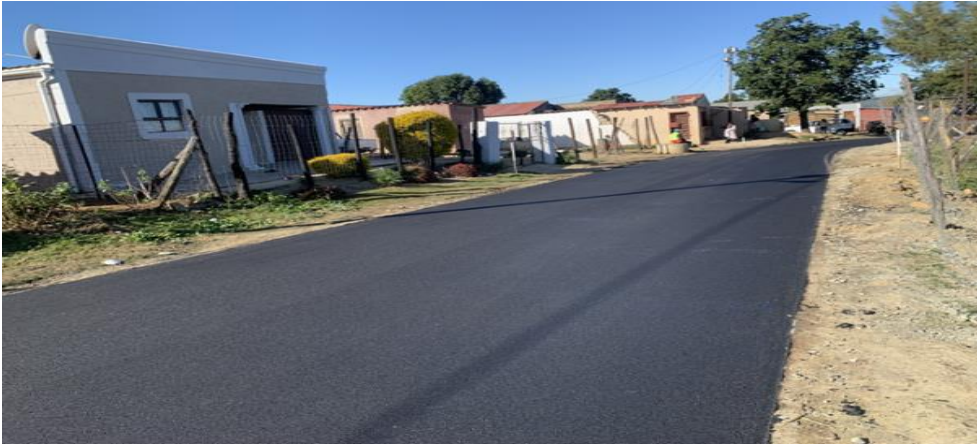
Image 6 - Urban Roads Upgrade and Rehabilitation – Phase 5 : Thubalethu – (R 7,446,918.08)
