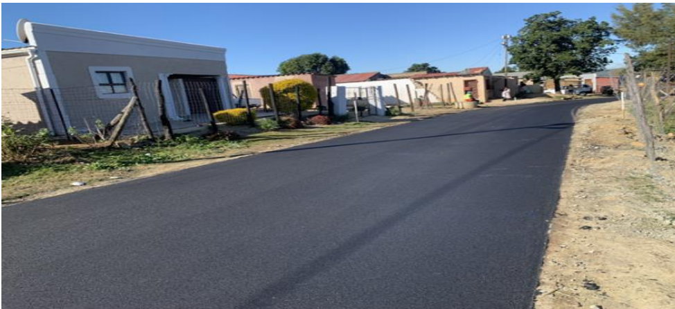
Image 27 - Urban Roads Upgrade and Rehabilitation – Phase 5 : Thubaletu – (R 7,446,918.08)
