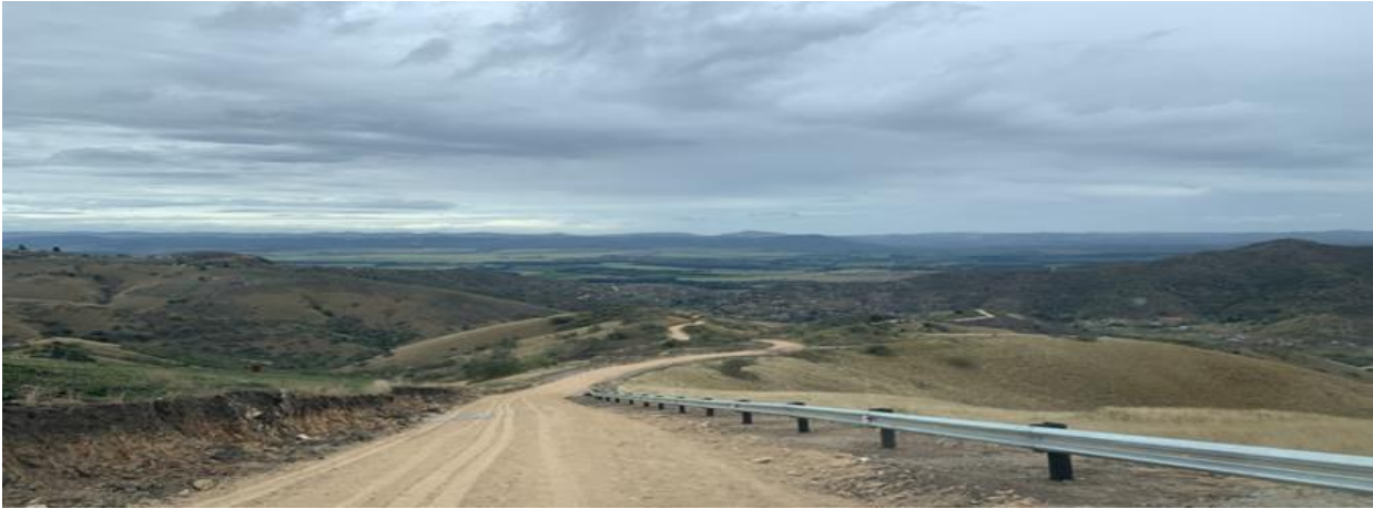
Image 4 - Makhubalo Gravel Road in Ward 9 – R 3,501,542.31
