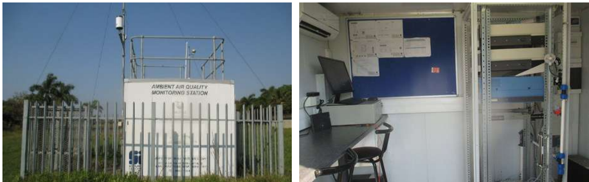
Ambient Air Monitoring Station
