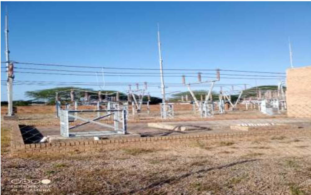
Picture :** Phoenix Substation 132/11kV 40MVA transformer installation: Ward 26; Co-ordinates: 28°43'27.1"S 32°02'04.0"E
