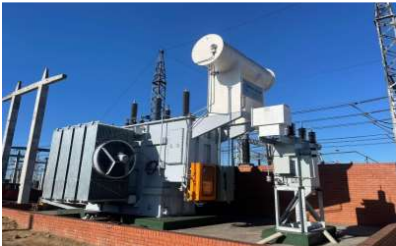
Picture **: Polaris Substation 132/11kV 40MVA transformers installation: Ward 2; Co-ordinates: 28°46'41.6"S 32°00'57.4"E
