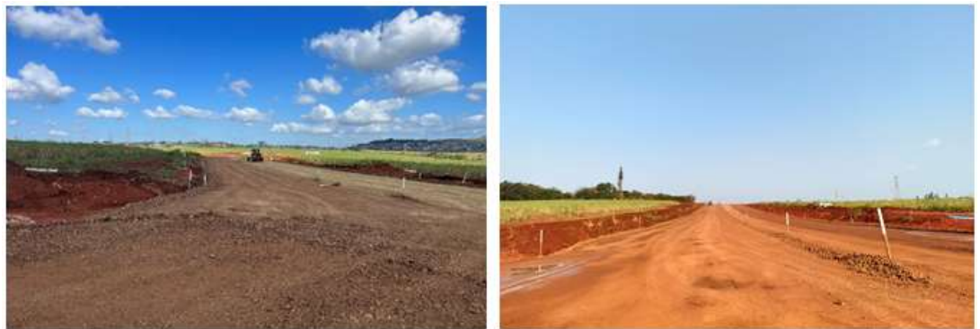
Empangeni Mega Housing Phase 3 Internal Bulk Construction
