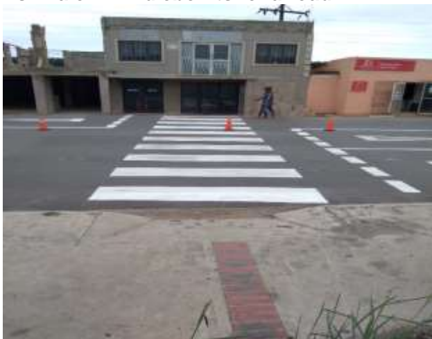
ROAD SIGNS INSTALLATION Western arterial road in Alton
