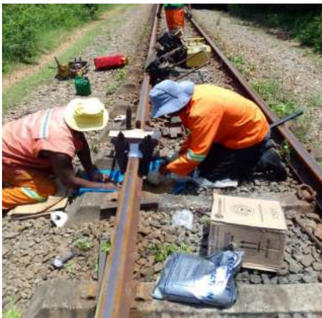
Railway line repairs (Siding No. PS 651613) Alton
