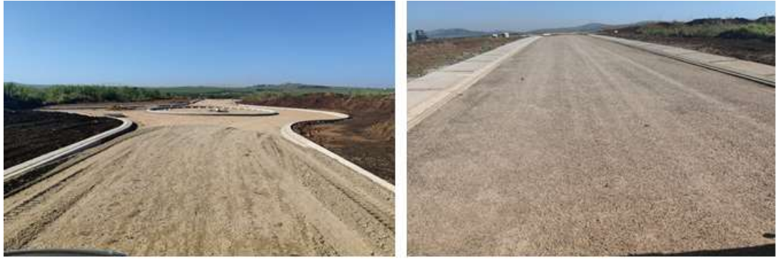
Empangeni Mega Housing Phase 2 Internal Bulk Construction
