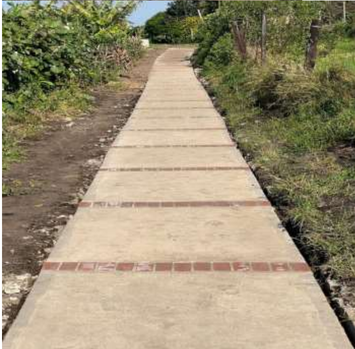
c. Construction of the walkway in Ward 22 Esikhaleni: Emoji Projects
