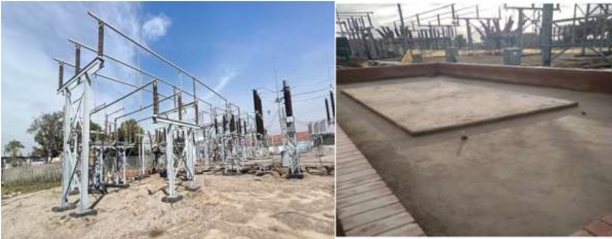
Picture :** Cygnus Substation 132/11kV 40MVA transformer installation: Ward 22; Co-ordinates: 28°53'09.0"S 31°54'02.5"E
