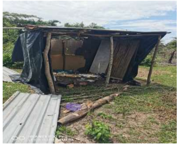
Illegal Structure identified and removed by Vagrant and Squatting control team
