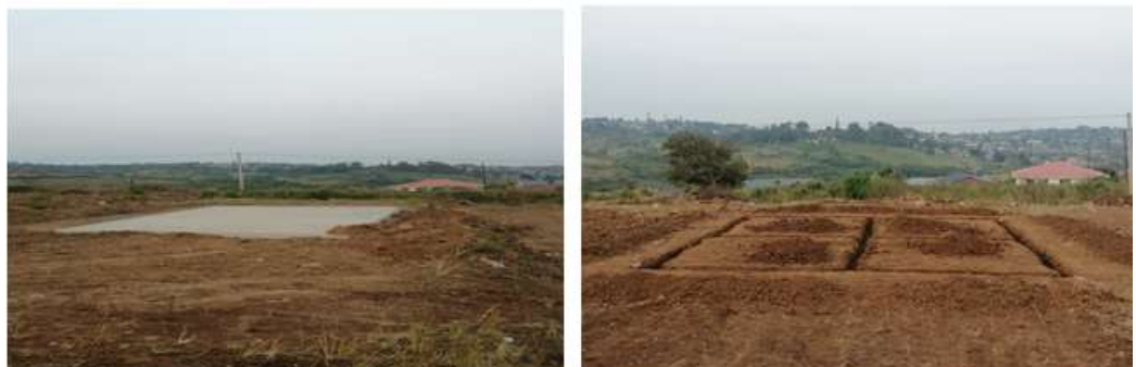
Dumisani Makhaye Village Phase 8 slabs
