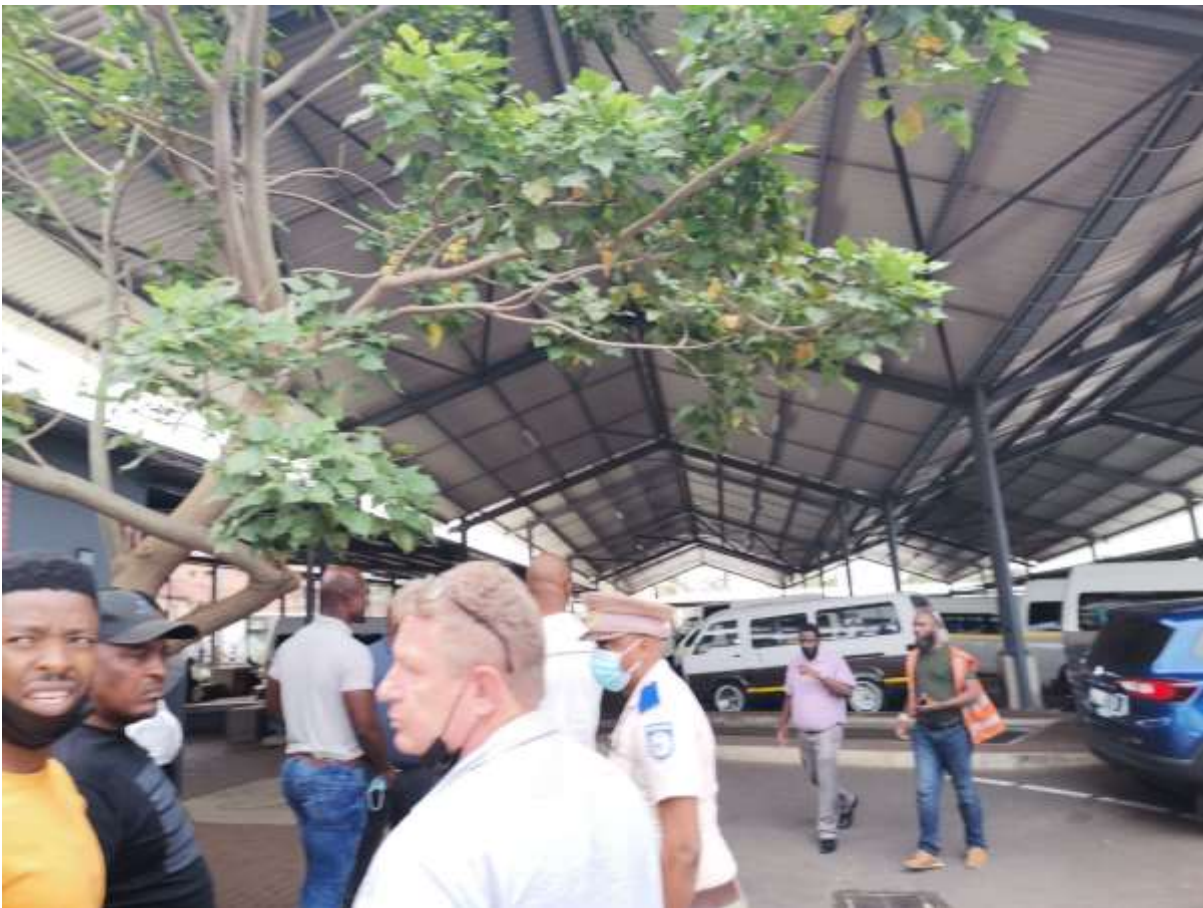
Site visit of the rank facility under Ethekewini Municipality
