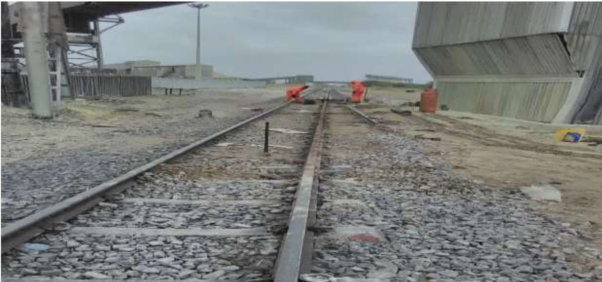
Welding at the Foskor Siding
