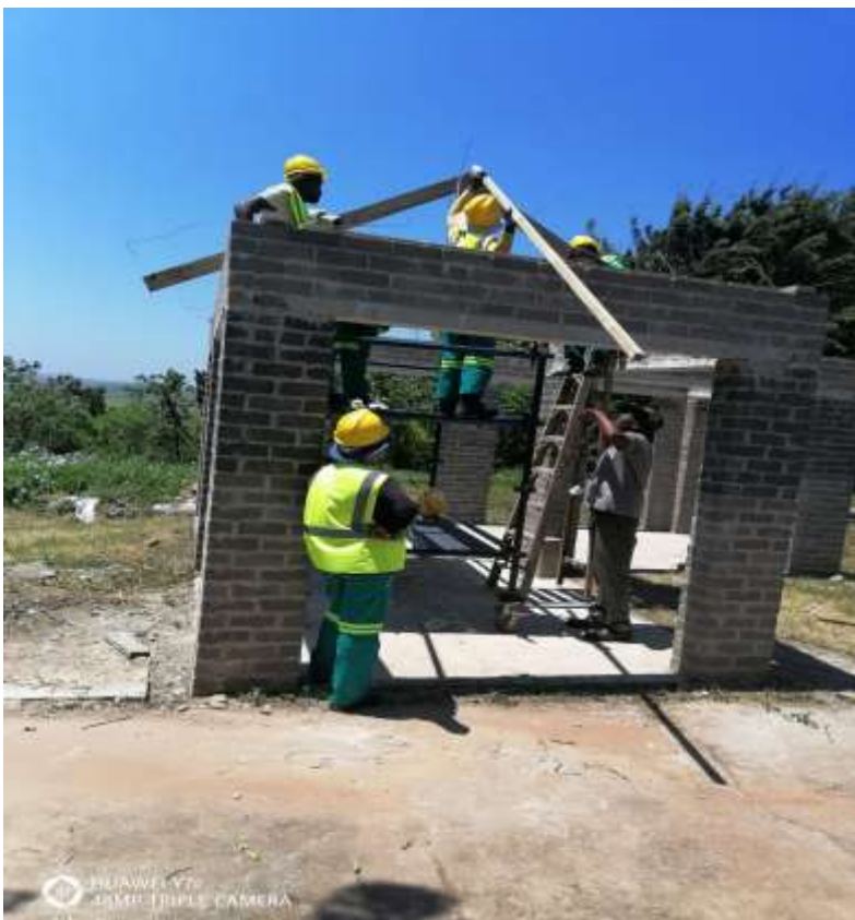
Figure 4: Basic building construction skills
