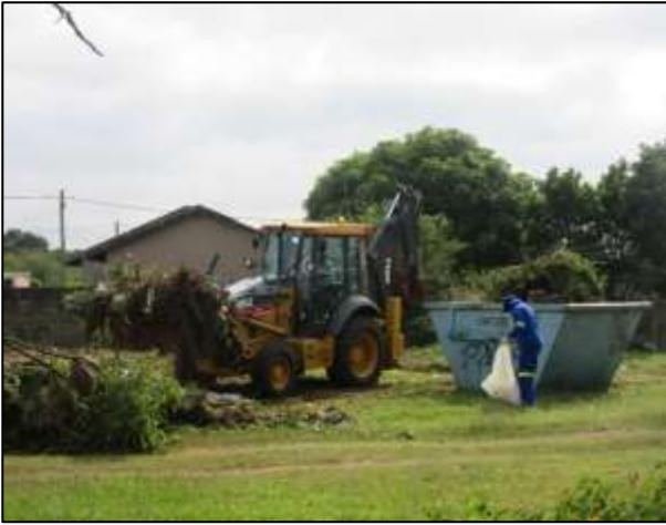
Ward 09 – Kildare illegal dump clean-up
