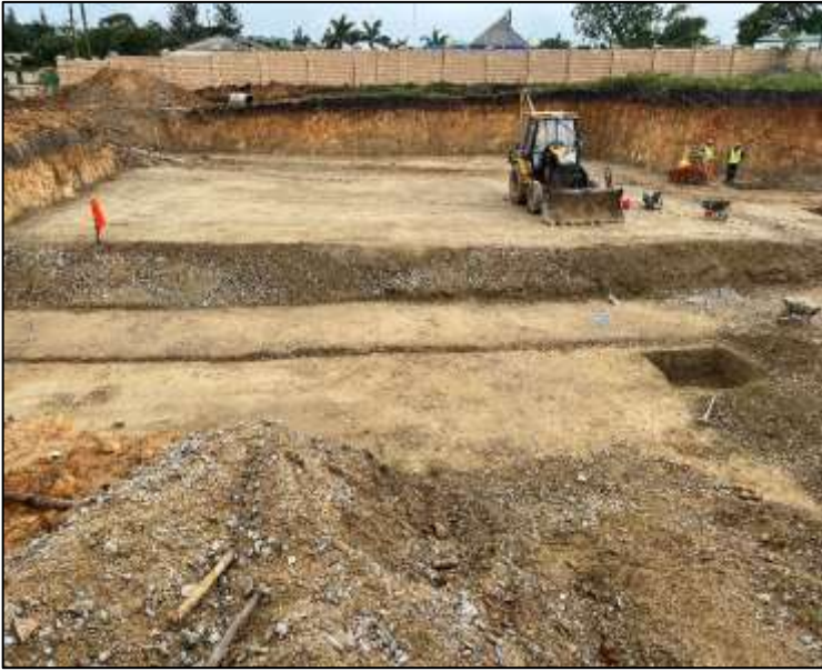
Earth works at the Kwadlangezwa swimming pool
