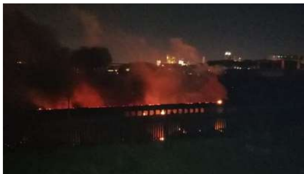
Electrician Fire at Scorpio Substation Empangeni CBD
