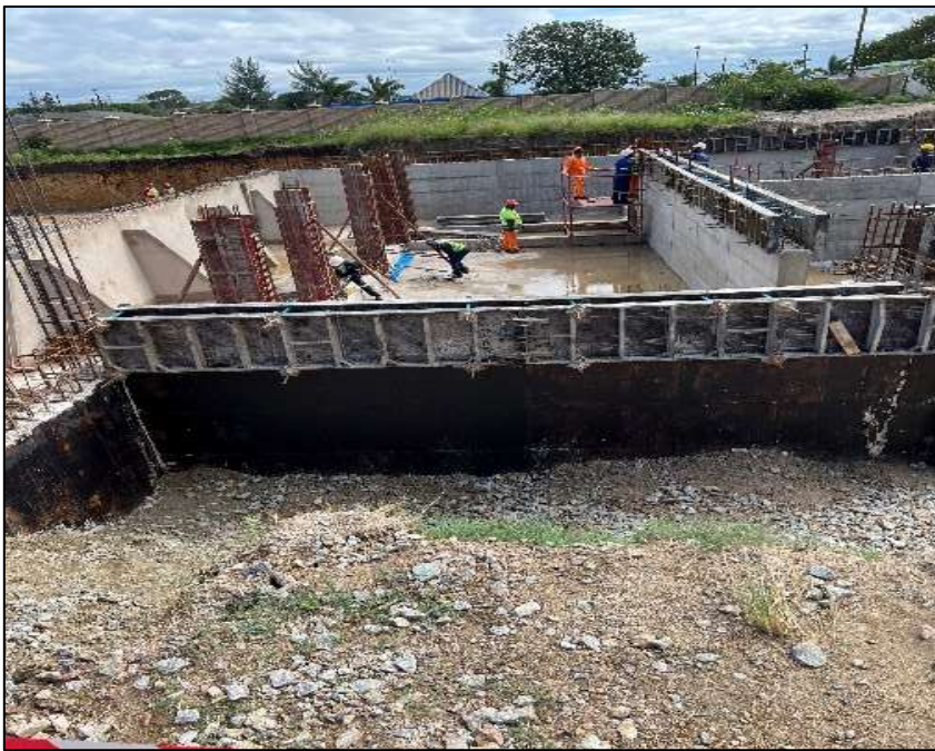
The completion of 3 parts of the Kwadlangezwa swimming pool wall.
