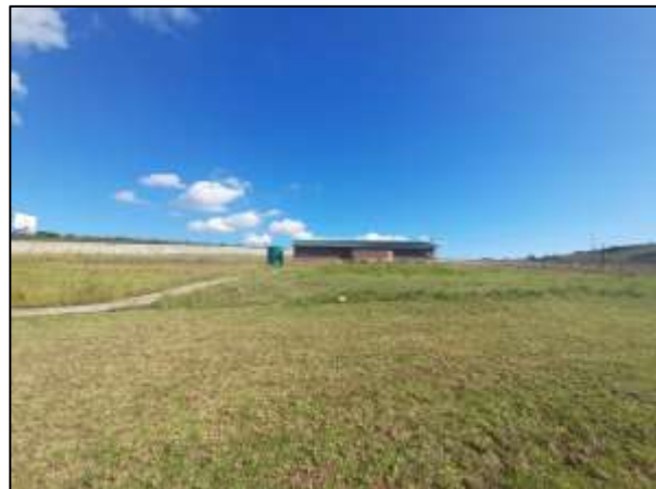
Ablution facilities at Madlebe Sport Field
